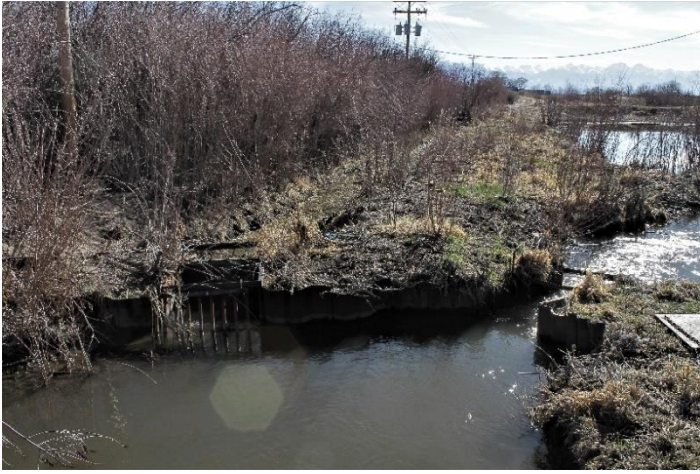
Headgate looking downstream
