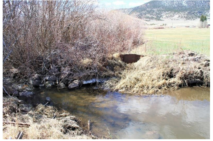
Headgate and diversion dam
