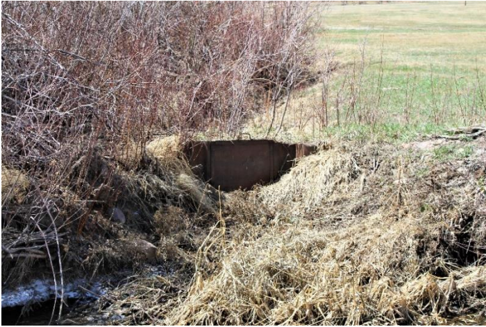
Headgate looking downstream
