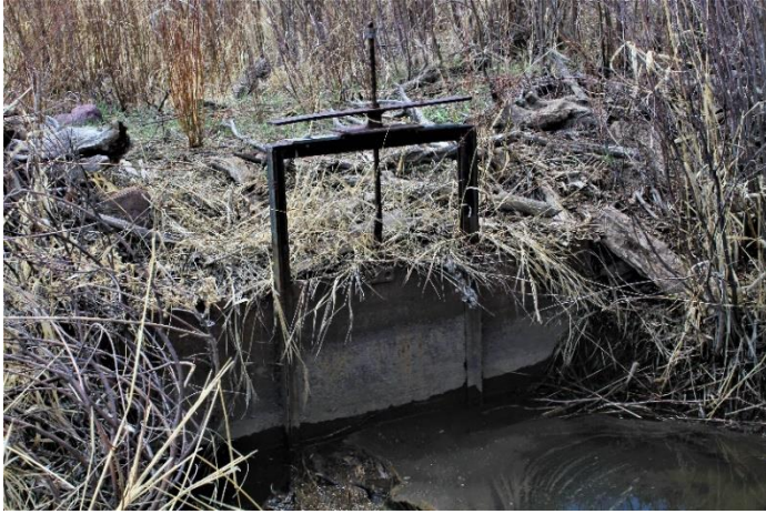
Headgate looking downstream
