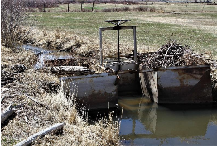
Headgate looking downstream
