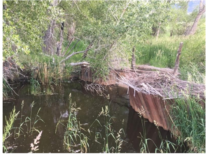
Diversion dam looking downstream
