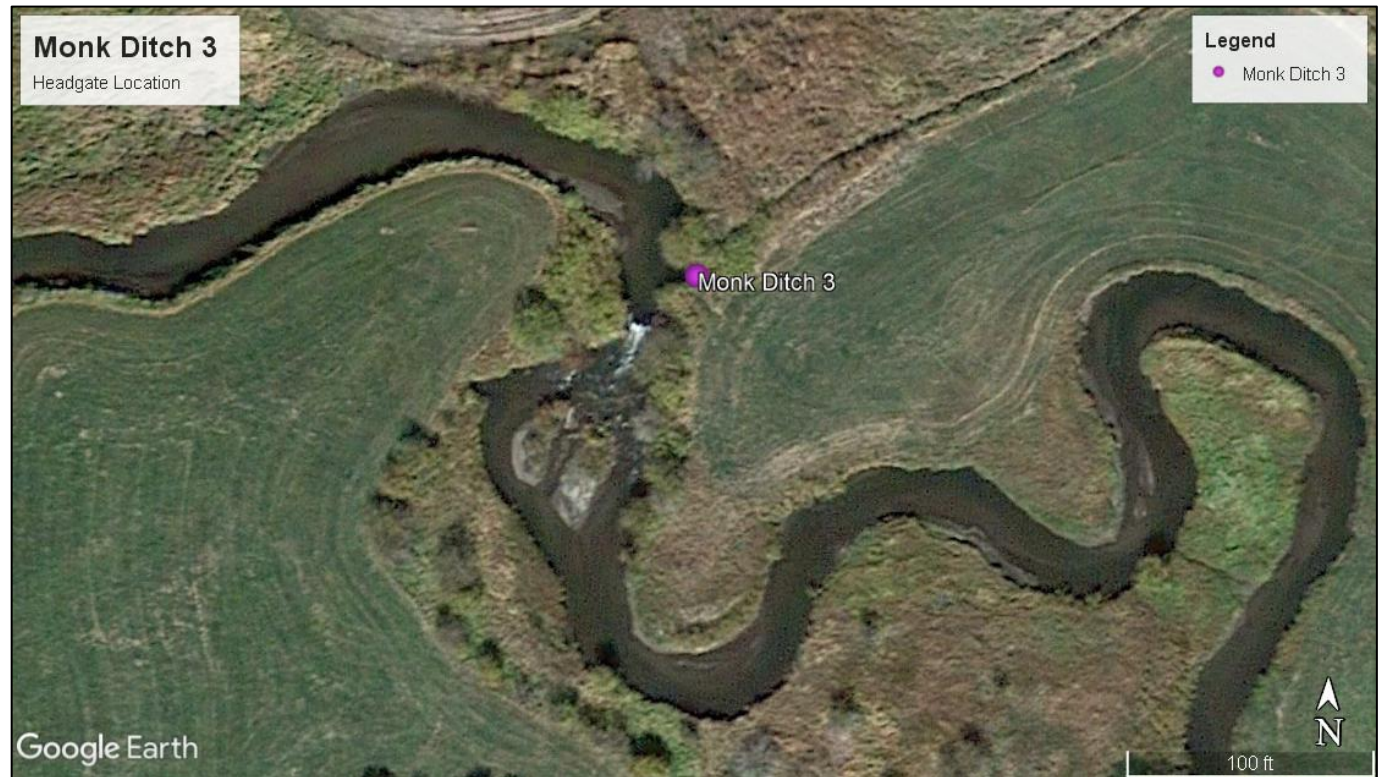
Close-up of headgate and diversion dam. This image illustrates the channel constriction caused by the diversion dam and resulting effects on the stream.
