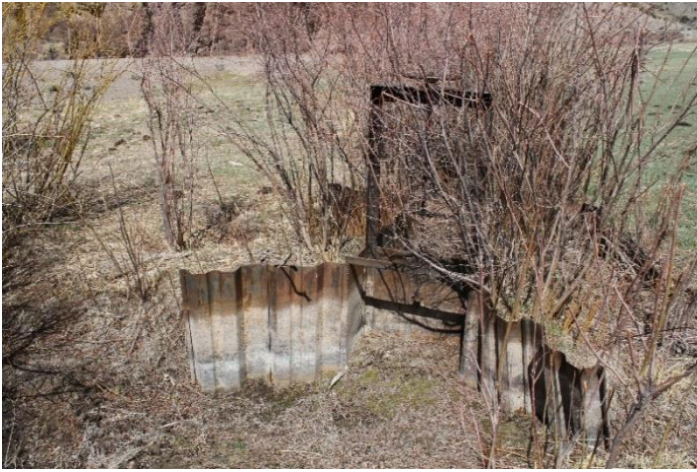
Headgate looking downstream
