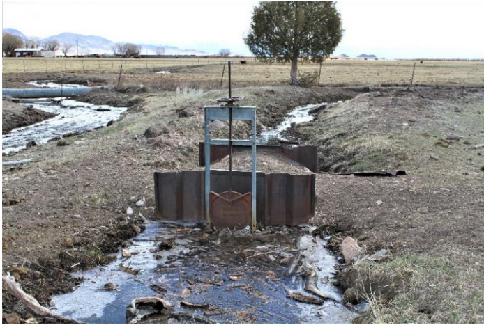
Headgate looking downstream
