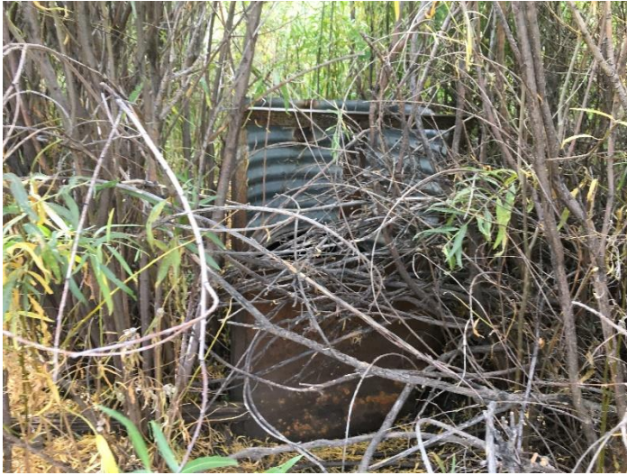
Headgate looking downstream
