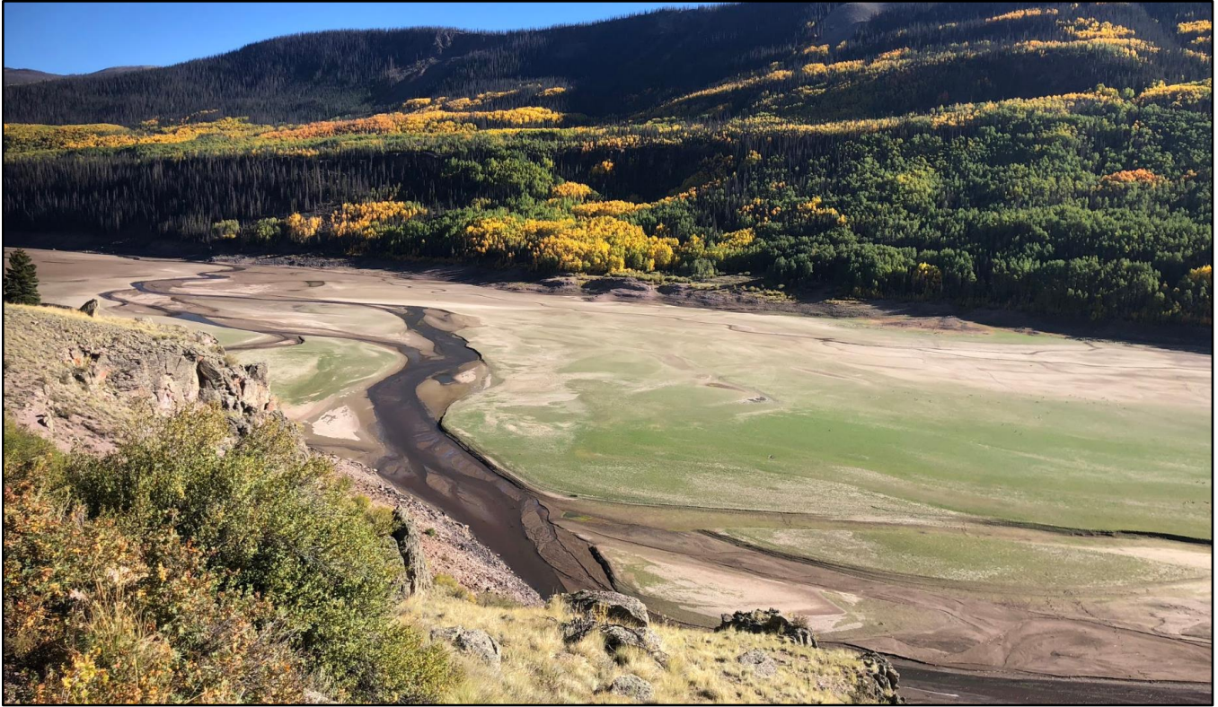
Figure 2.17: Sediment trapped behind the Rio Grande Reservoir (seen during dam repairs which had the reservoir drained during the fall of 2018).
