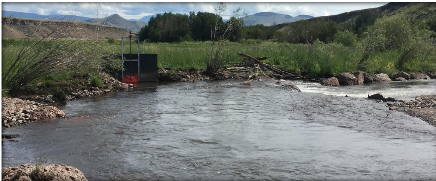
Figure 4.1: Middle D-Curtis Ditch diversion and headgate on Saguache Creek.
