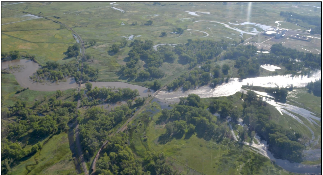
Figure 2.13: Railroad lines and bridges crossing the Rio Grande near flood stage, June 2019.
