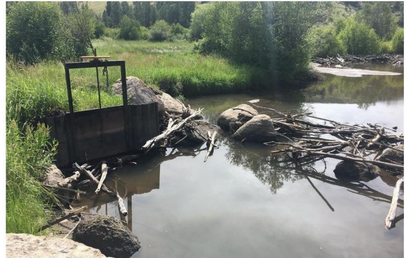
Headgate and diversion looking downstream
