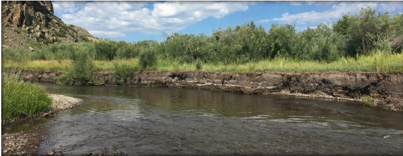
Figure 4.2: Bank and channel instability downstream of the Middle Creek confluence.
