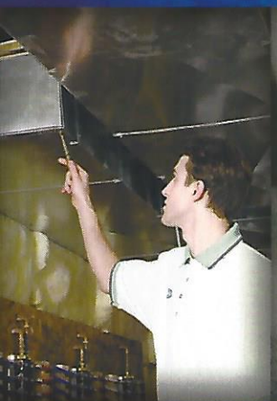
AeroSeal technician conducts initial diagnosis by analyzing airflow
