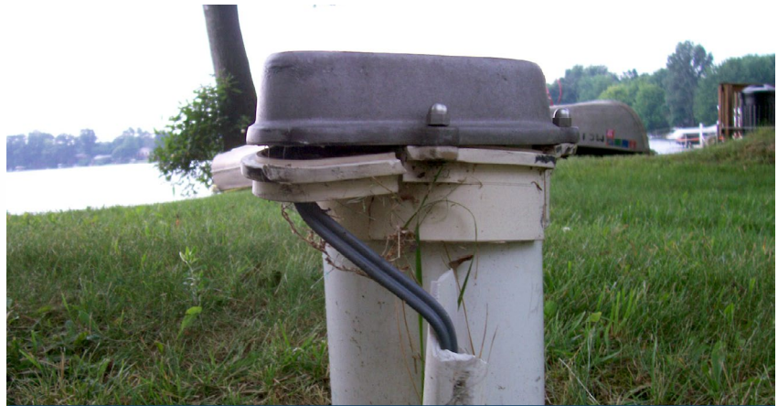
Damaged wellhead with cracked well cap and exposed wires
