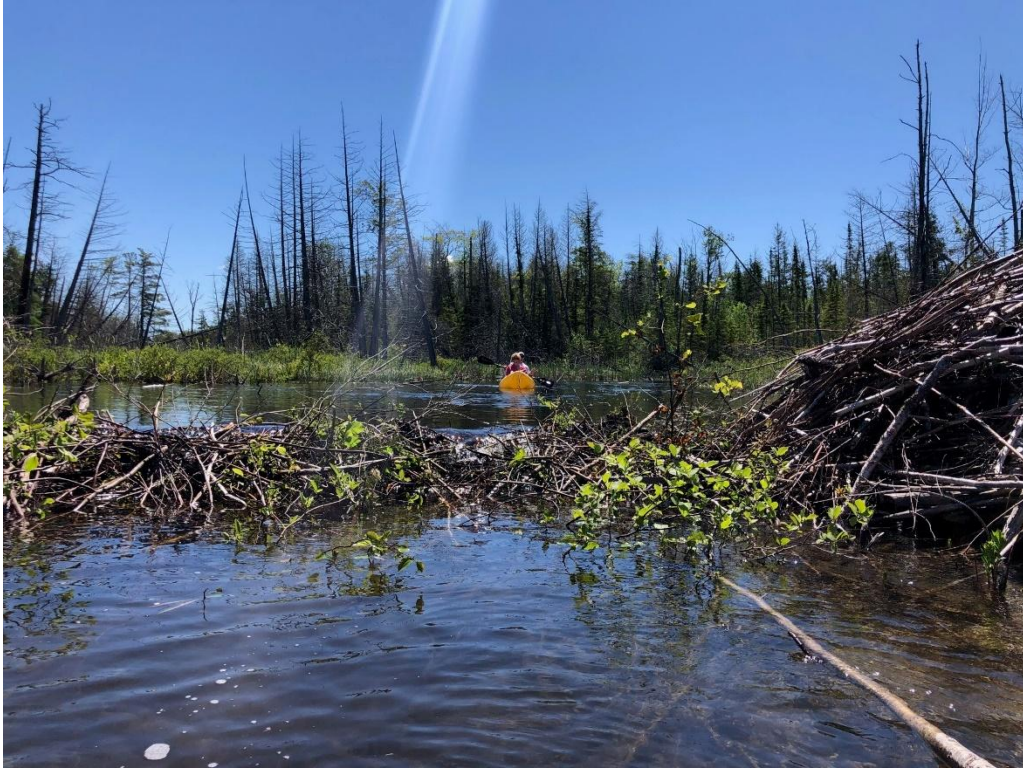
2 - Dam between Little Traverse Lake / CR669 prior to removal June 2020
