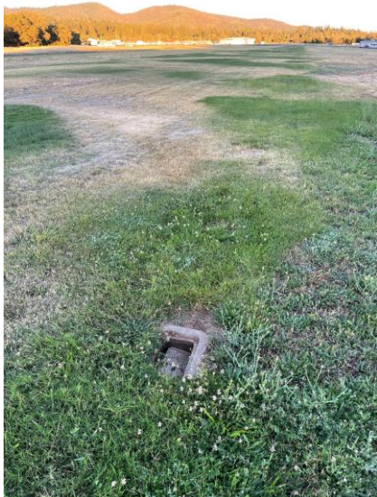
Open irrigation hole on runway 29. No action has been taken to repair the hazard since June.
