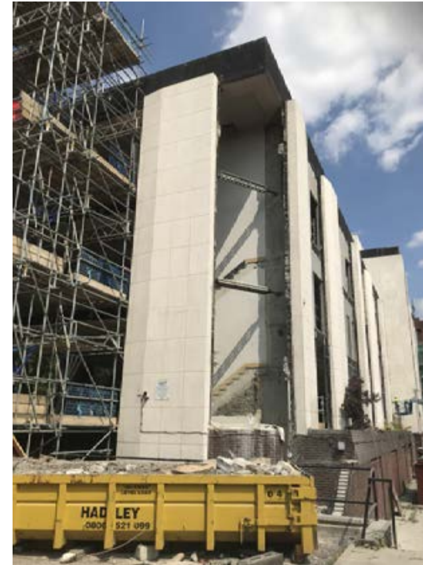
Pre-Installation East & West Staircores
