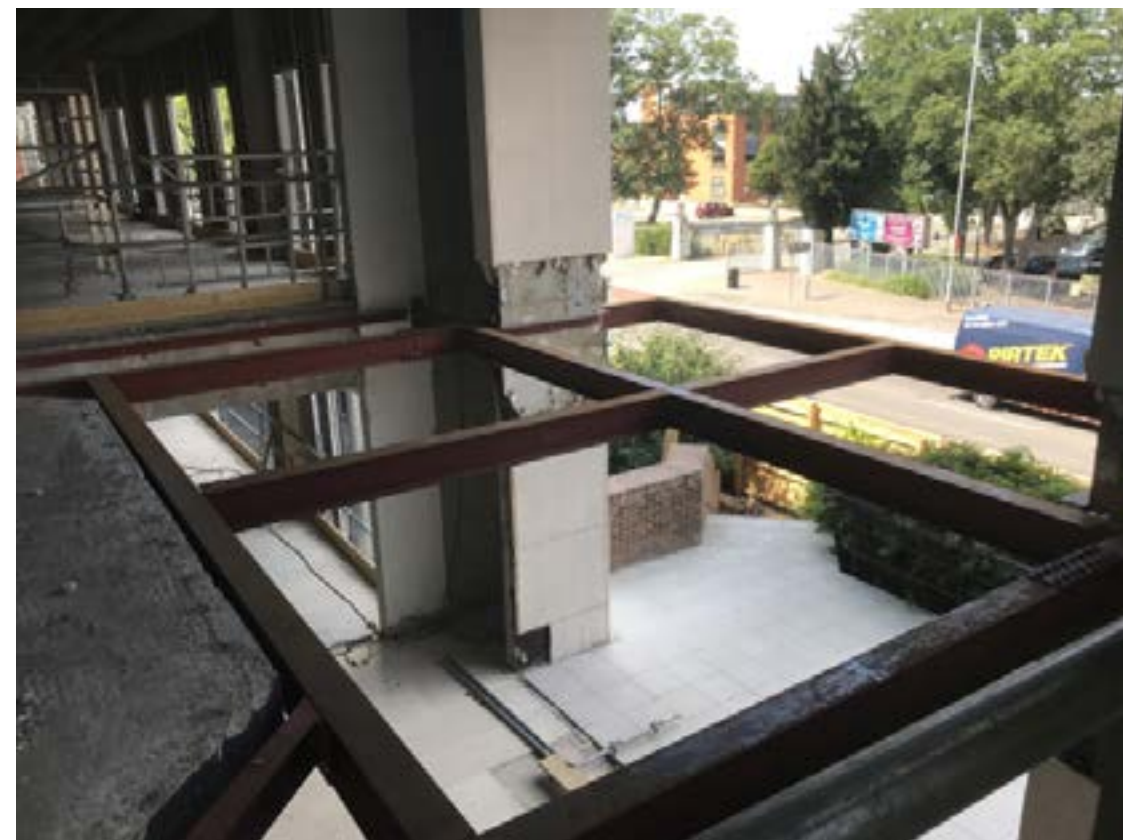
Post Installation Lobby Area
