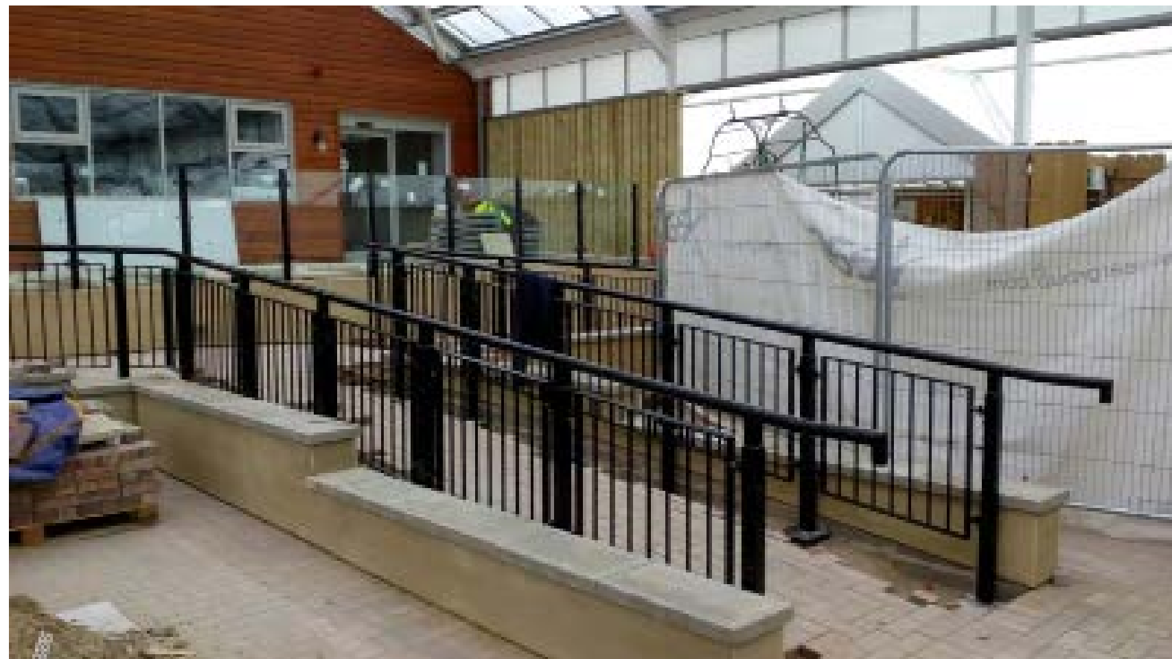
Pedestrian Ramp Railings & Glass Balustrading to Restaurant Patio
