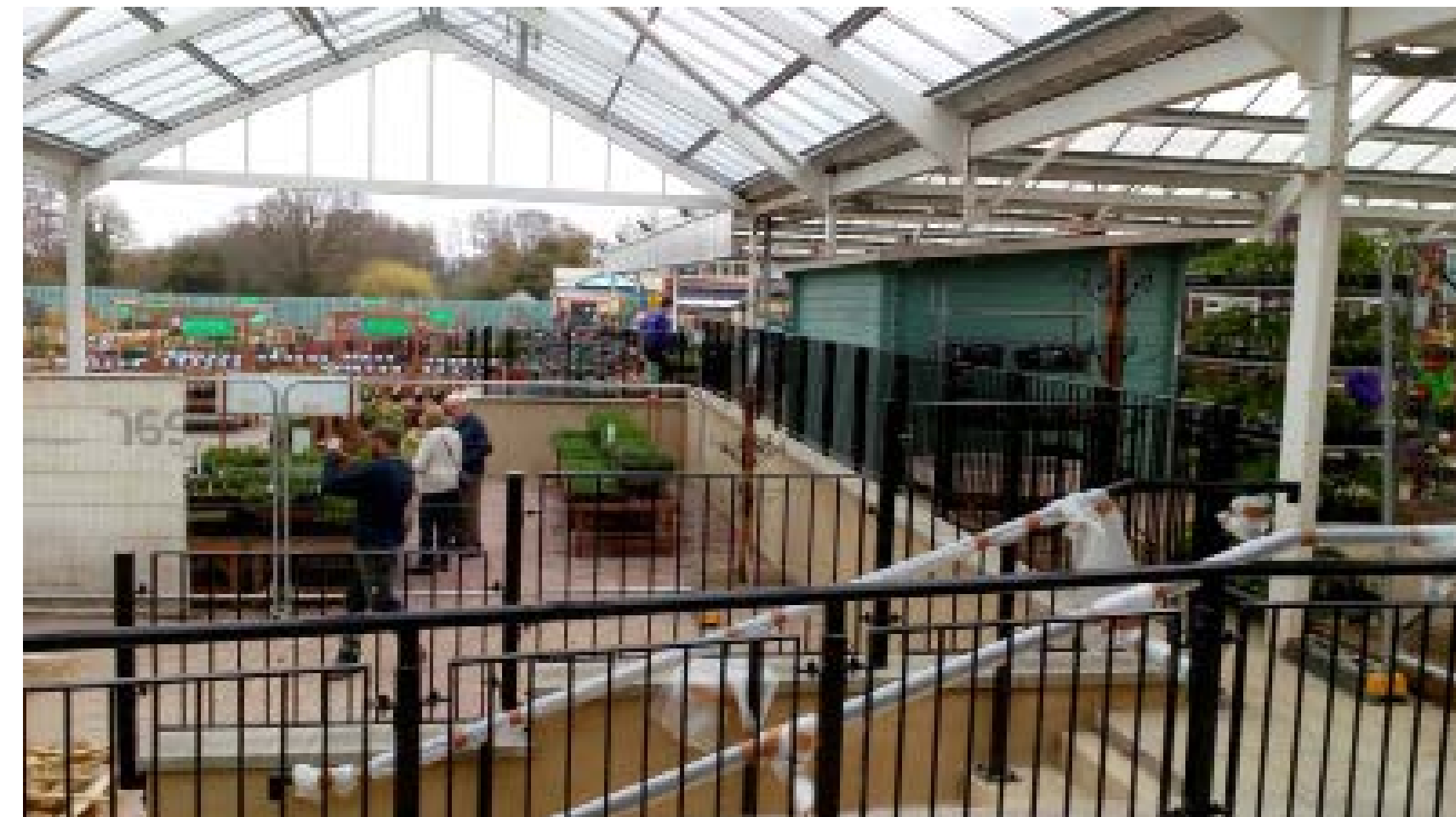
Railings to Stairs and Raised Platform
