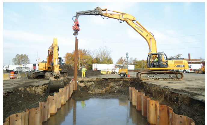
Everett Emergency Culvert Repair at Boston New Market Terminal (2012)
