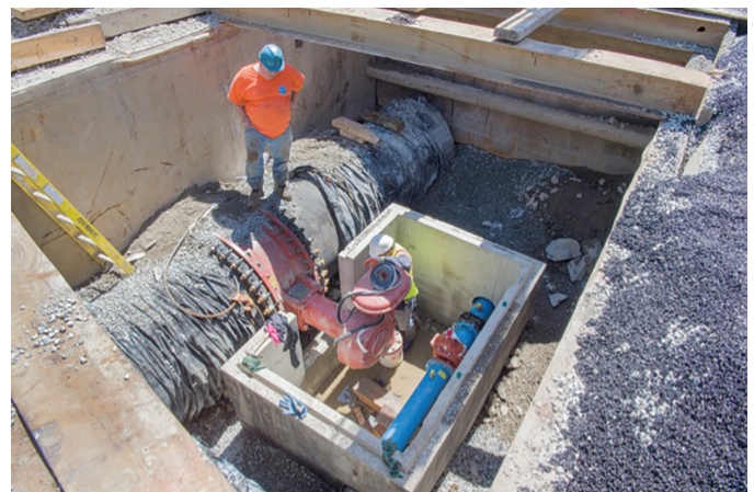
Installing 48-inch butterfly valve and vault on Route 28.
