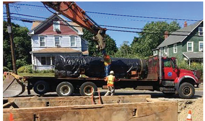
Trailer delivering 48-inch pipe with poly wrap to crew.
