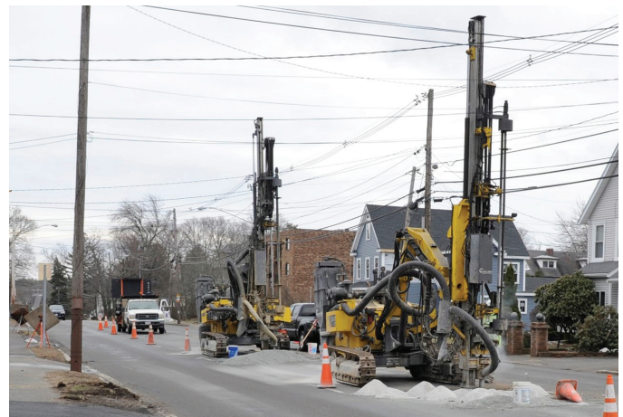
Predrilling rock on Main Street
