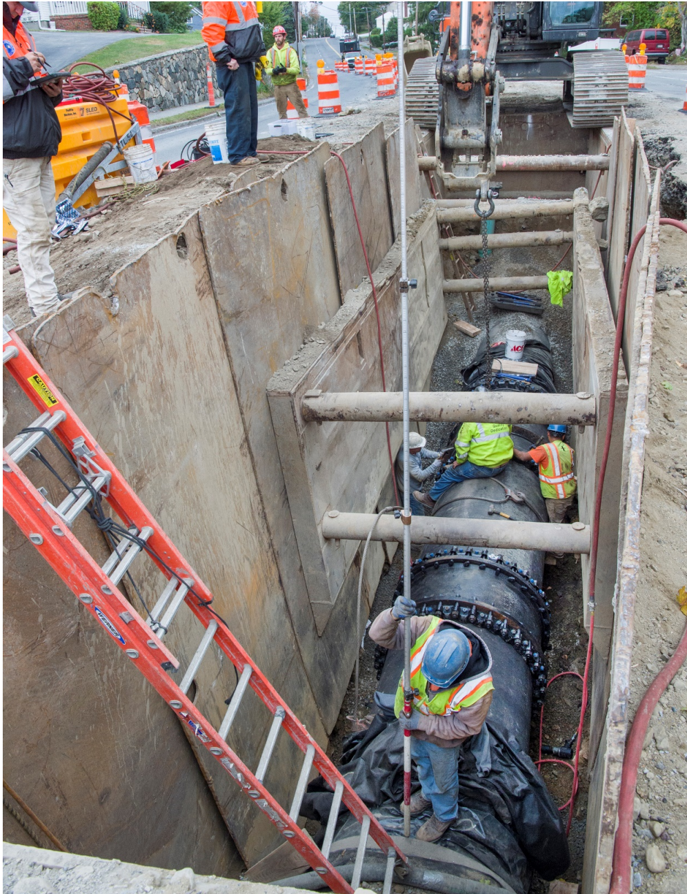
Connection of 48-inch pipes on Main Street
