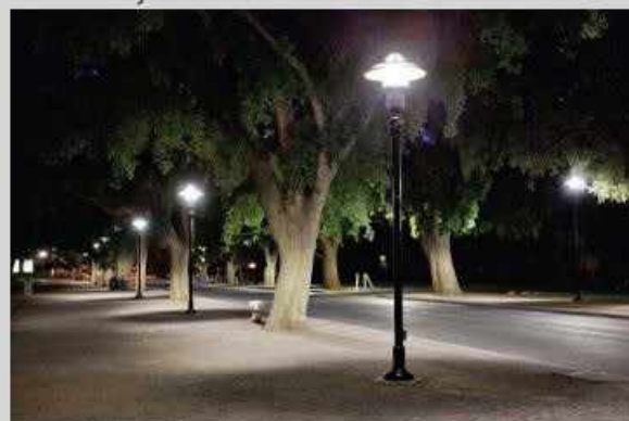
Lights that are down lit and/or utilizing shields help to reduce glare and light pollution. These are preferred instead of typical acorn light fixtures.
