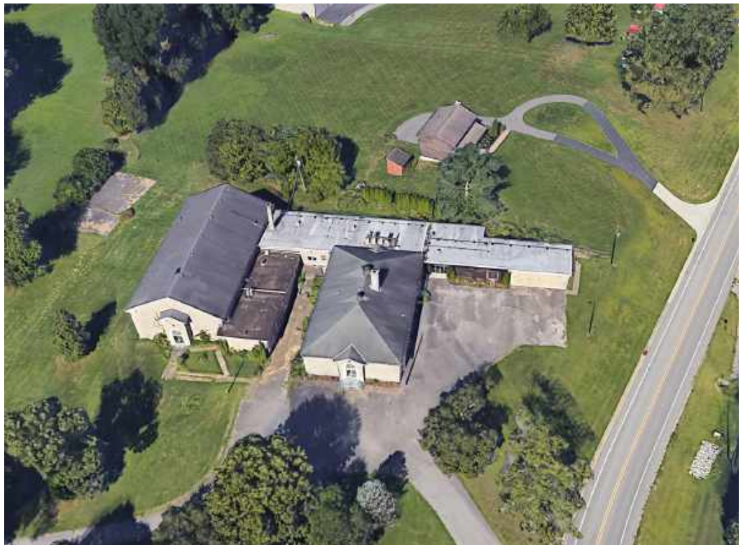
The old Utica Elementary School building off Old Salem Road has the opportunity to be redeveloped and renovated as a community and civic center for the Town.
