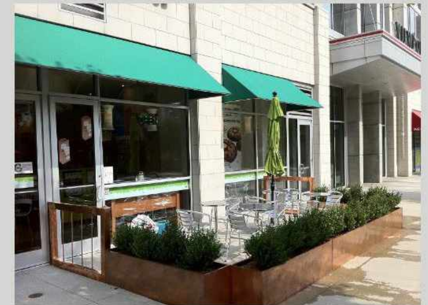
Planters, as seen in the picture above, can be wonderful tools to help differentiate the foundation of a building from a large sidewalk. This creates a more intimate feel for patrons while also adding a dynamic visual improvement to the surrounding area by introducing leafy materials in an otherwise very harsh environment.
