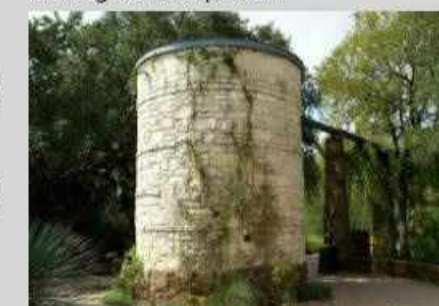
Water cisterns capture rainwater to reuse on irrigation or as grey water.
