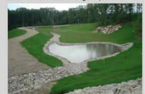
Retention ponds will reduce the flow of stormwater and filter out pollutants.
