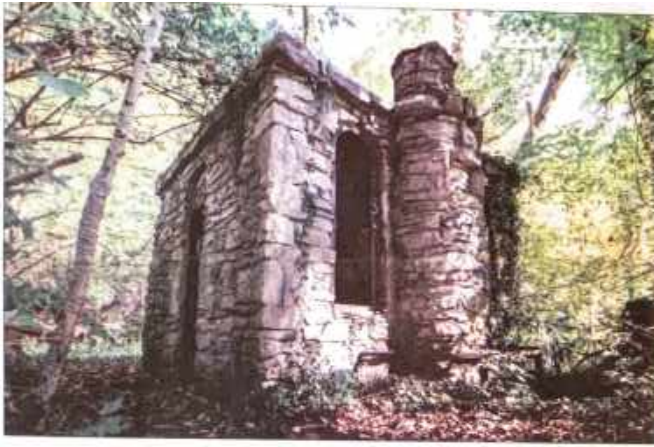
This file photo from 2017 shows a stone structure up the hill from the ruined foundation of the Witches' Castle. Photos and Tribune File
