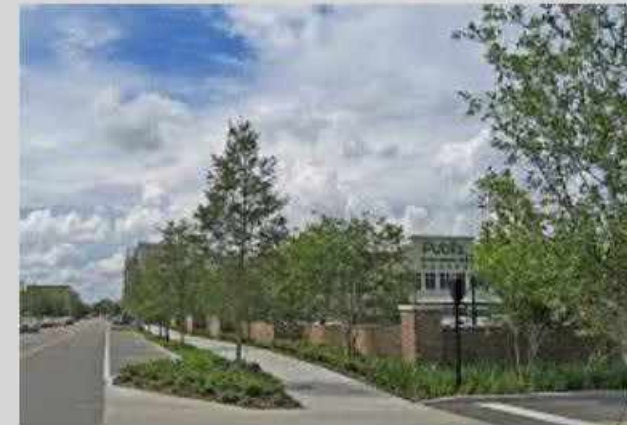
A large amount of parking is shown with the building still in front of the lot with parking screened and located to the side.
