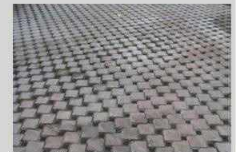
Permeable pavers reduce stormwater runoff rate and recharge aquifers.
