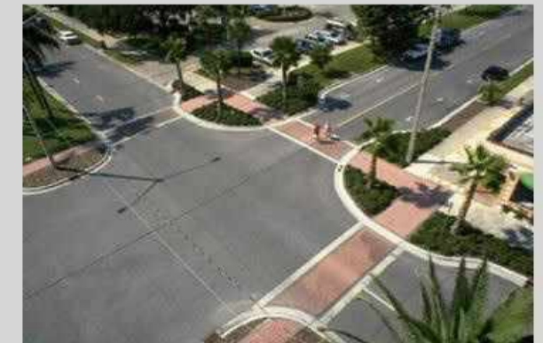
Bump-outs extend the curb outward in order to narrow the street and make drivers pay more attention while also placing pedestrians more in their line of sight.
