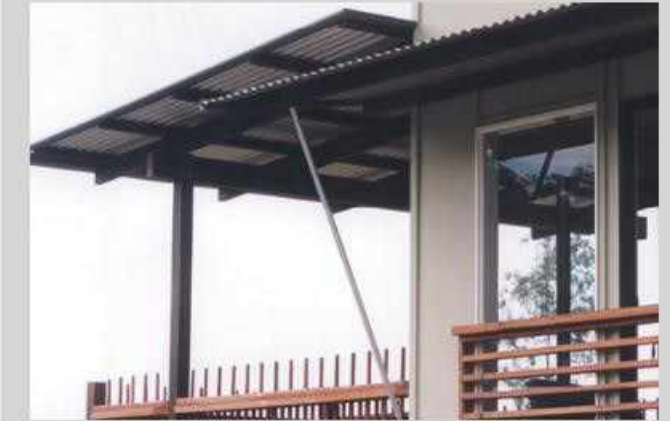
Sun shading devices can be used to reduce solar heat gain and provide visual interest.
