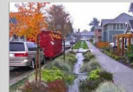
Bio-swales to filter water and recharge underground aquifers.
