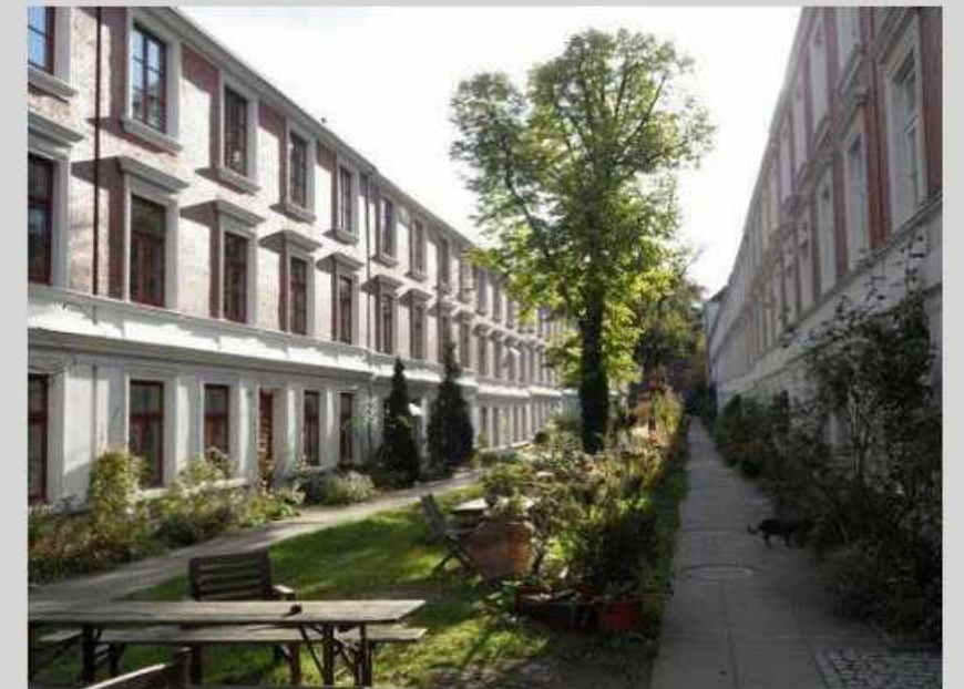
Adding foundation plantings to areas between residential buildings creates dynamic public spaces for children to play, for people to walk their dogs, and for neighborhood gatherings. The example above shows a space between two apartment building that uses foundation plantings to create a dynamic community space, as opposed to the typical parking lot or through street.
