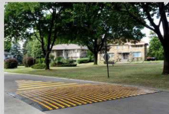
Speed tables are becoming increasingly popular as methods of traffic calming in residential areas, as they are much larger and have a more intense slope, thus greatly reducing speeds.
