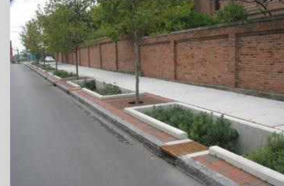
Rain gardens or bio-swales along roadways creates an interesting visual effect and allows for reduced environmental impacts of water on-site.
