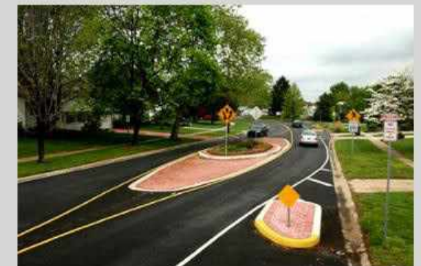
Traffic islands adjust the alignment of the curb forcing drivers to turn the car slightly and pay more attention. These should incorporate vegetation to add visual appeal.
