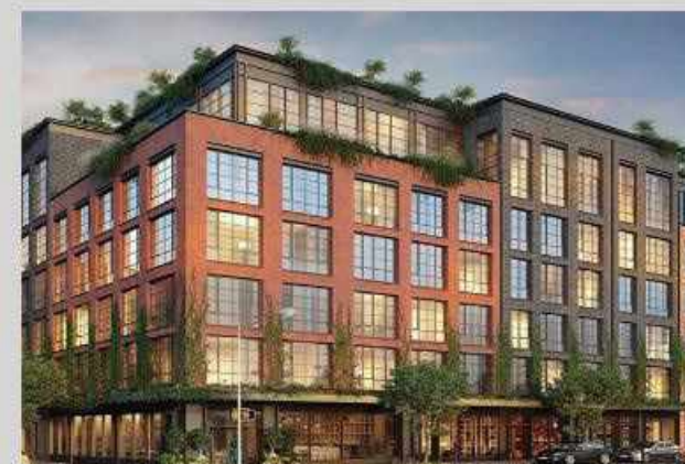
A diverse palette of materials will make for a vibrant district. Material selection should be sensitive to the context.
