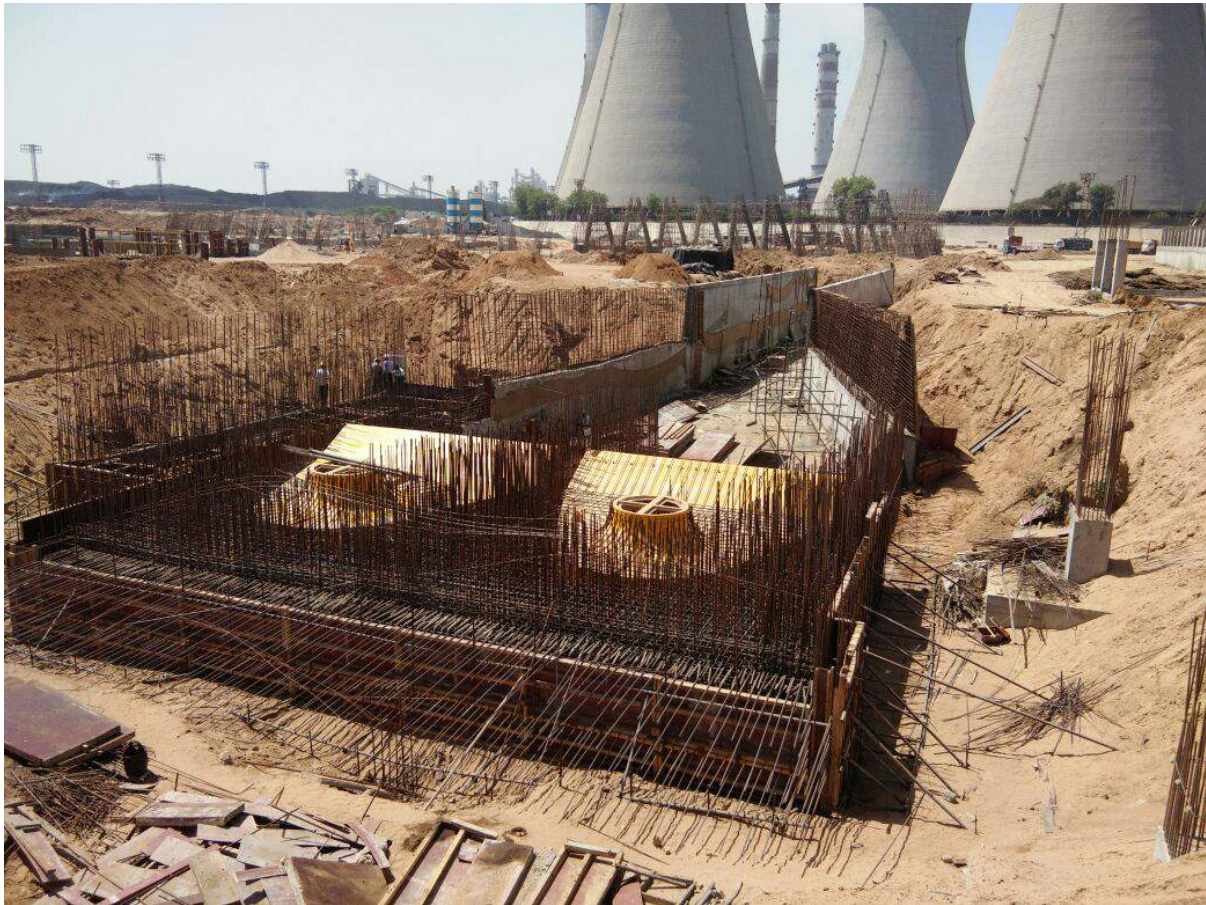
Concrete Volute Pump for 1x800MW Unit#8 Wanakbori Thermal Power Plant, Distt:-Kheda, Gujarat.
