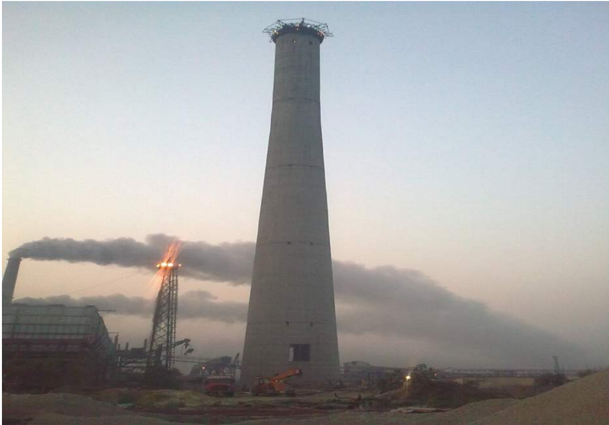
220 Mtrs high RCC Chimney at Harduaganj, Kasimpur, Distt:- Aligarh (U.P).
