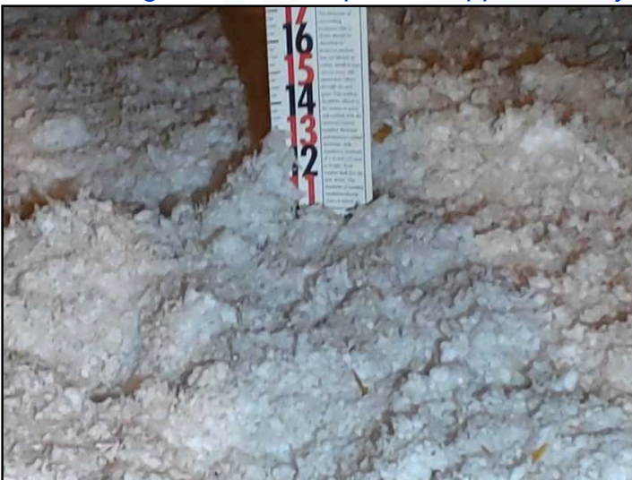
Average visible attic insulation depth was measured at 10 inches.
