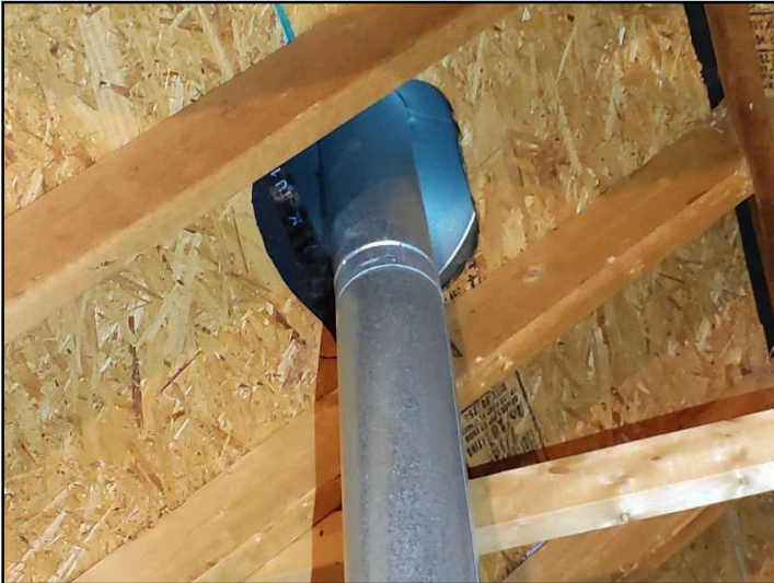
Underside of roof penetrations in attic
