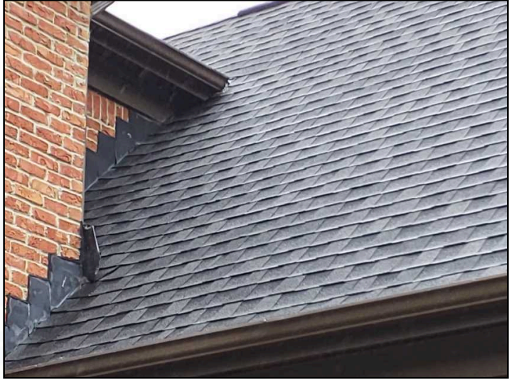
Roof covering image
