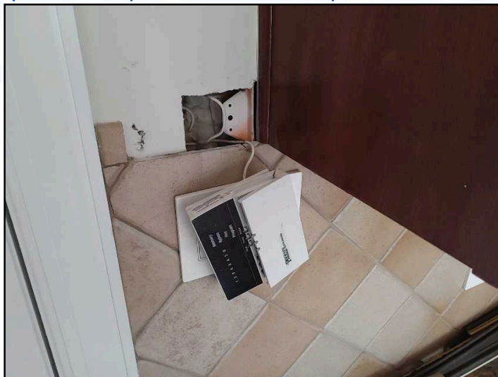
Any present Security systems are excluded from this inspection. Due to the specialized nature of these systems, we suggest that you review this system with the seller. As per our Inspection Agreement, this system is beyond the scope of this report and is not inspected.
