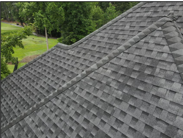
Roof covering image
