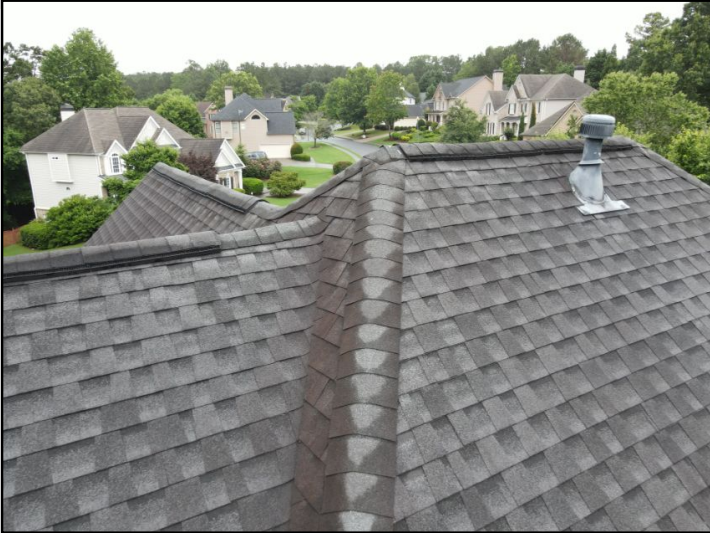
Roof covering image
