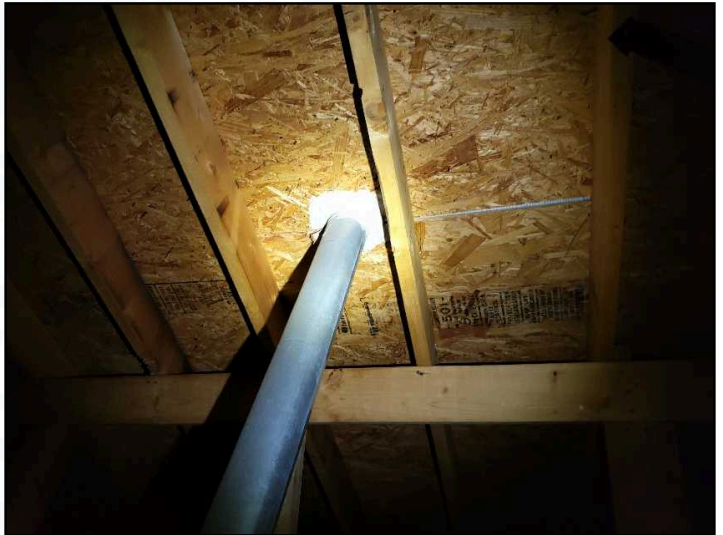
Underside of roof penetrations in attic
