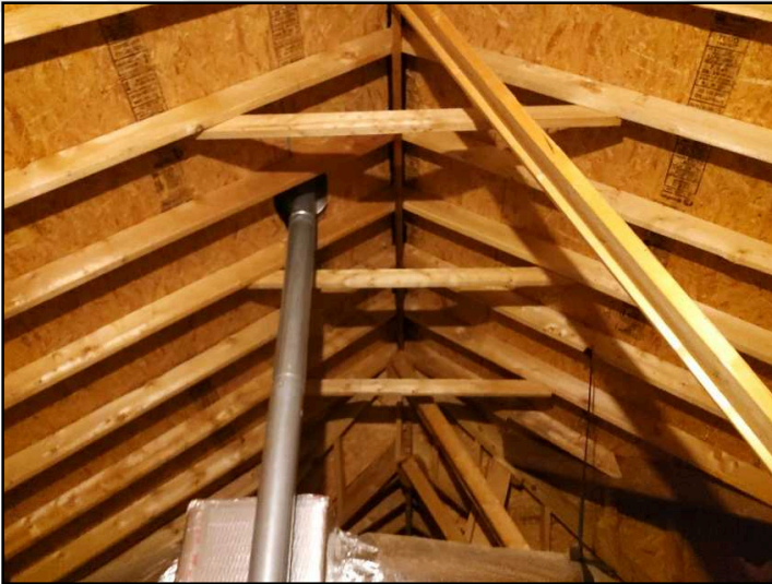
Attic framing image
