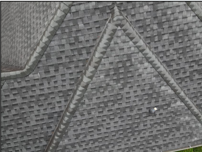
Roof covering image
