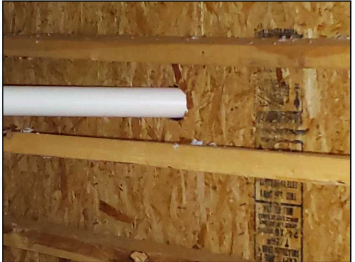
Underside of roof penetrations in attic
