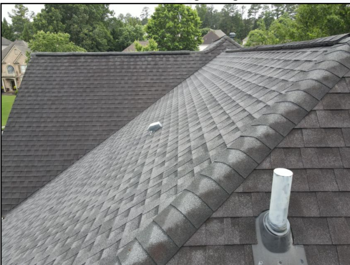
Roof covering image
