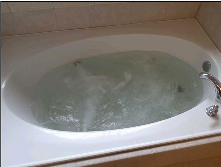
Jetted tub filled and briefly tested
