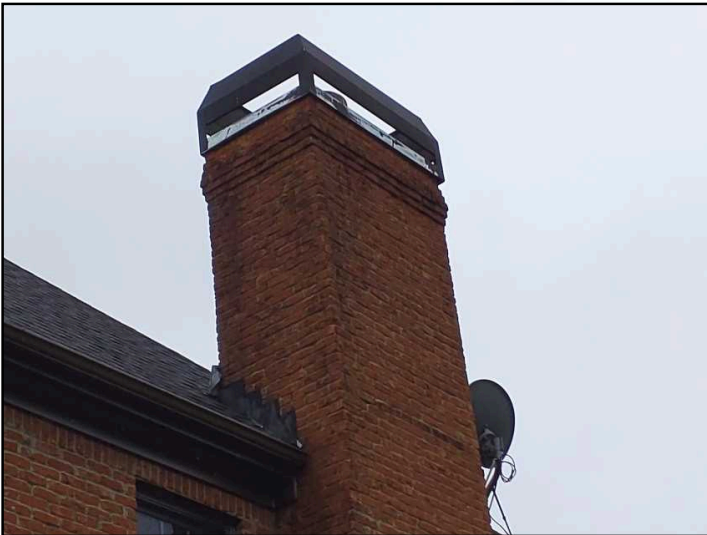
Horizontal and step cracking observed at exterior portion of chimney in brick veneer on right side of home near connection to gutter. Recommend further evaluation by qualified contractor to ensure structure of Chimney is not leaning or compromised and repair brick to prevent water intrusion
