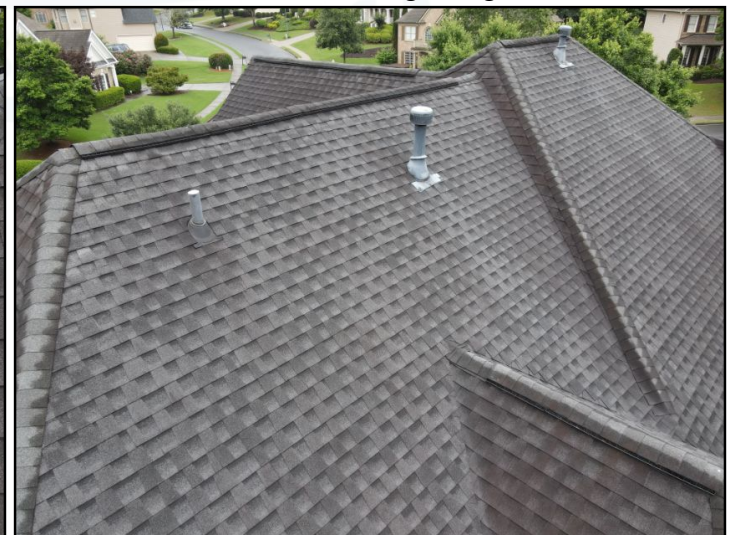
Roof covering image
