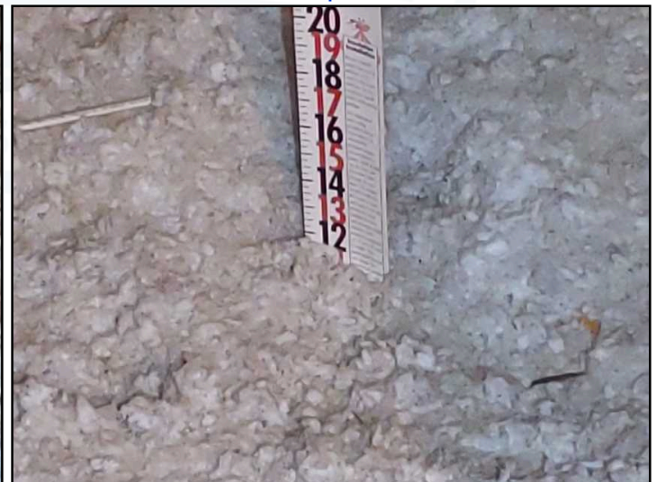
Average visible attic insulation depth was measured at 10 inches.
