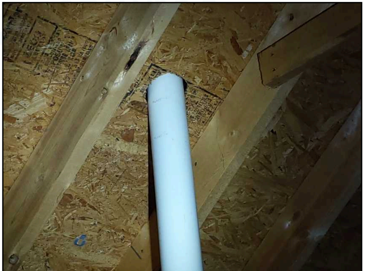
Underside of roof penetrations in attic
