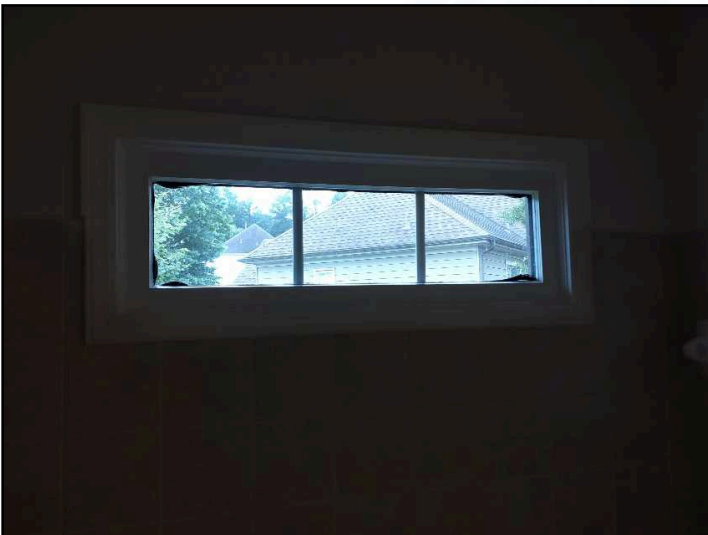
Warped/bulging seals noted at window above Jack and Jill bathtub
