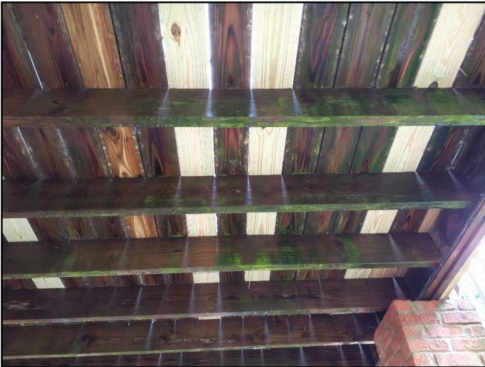
Underside of deck image
