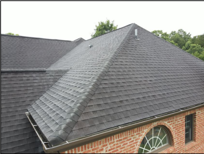
Roof covering image
