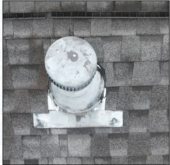
Roof penetration flashing image.
