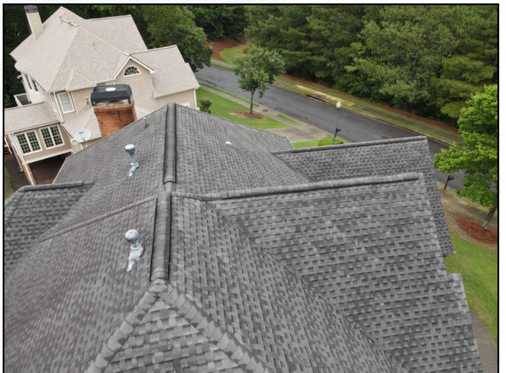
Roof covering image
