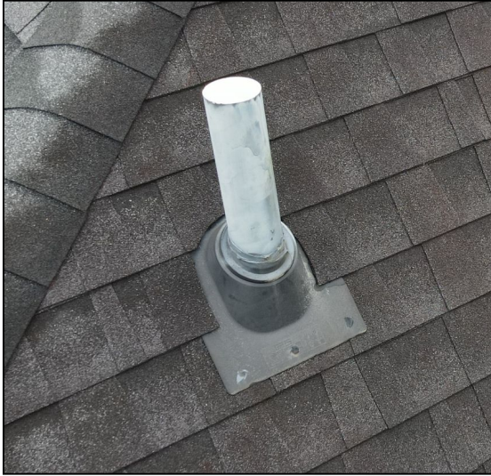
Roof penetration flashing image.
