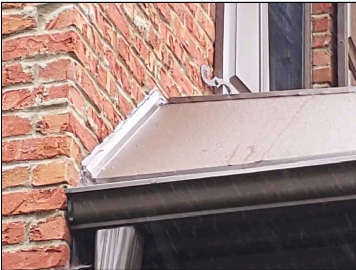
Roof covering image
