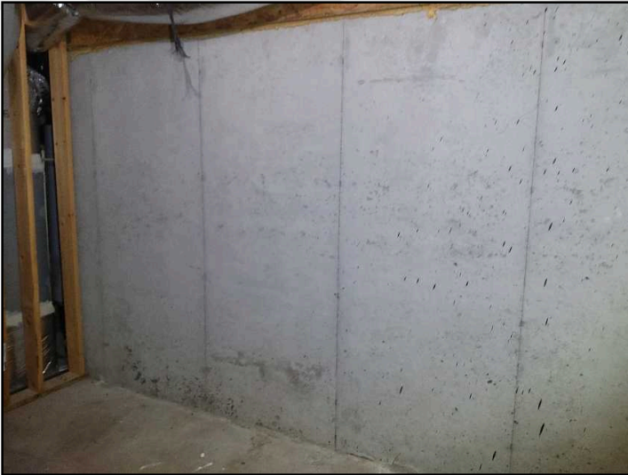
Foundation wall image
