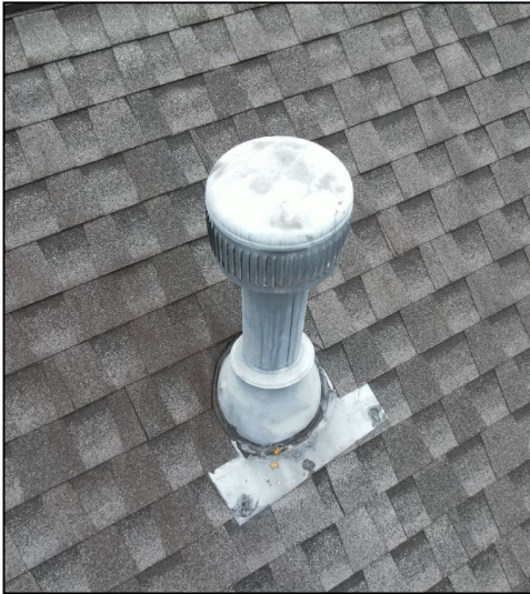
Roof penetration flashing image.
