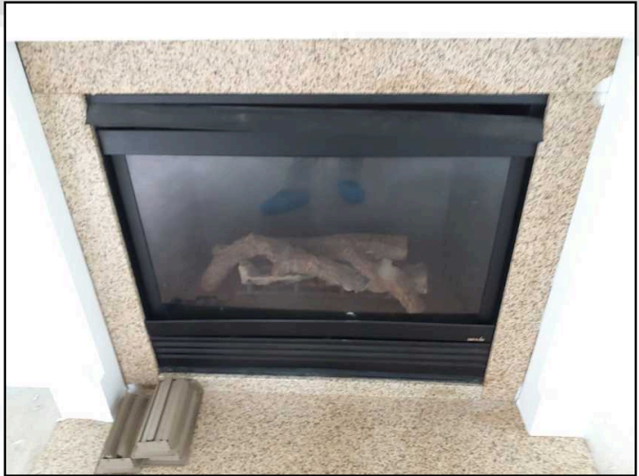
The gas line valve/pilot was shut off at the time of inspection.
