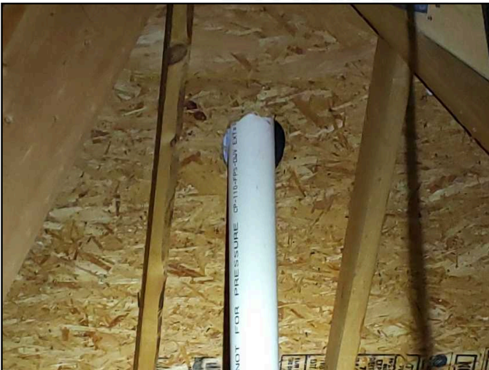
Underside of roof penetrations in attic
