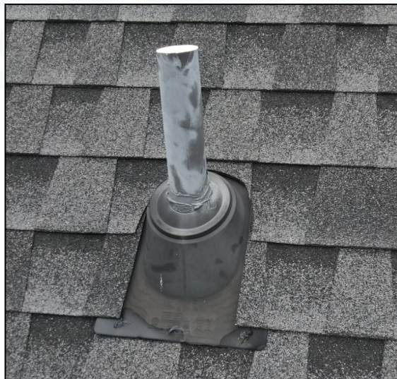
Roof penetration flashing image.
