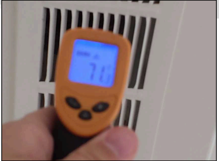
There was a 12 degree temperature differential when the air conditioning was tested at the upper floor level.
