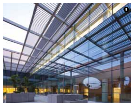
8 Champalimaud Centre for the Unknown, Lisbon, Portugal The Helvar router also controls all the blinds inside the buildings.
