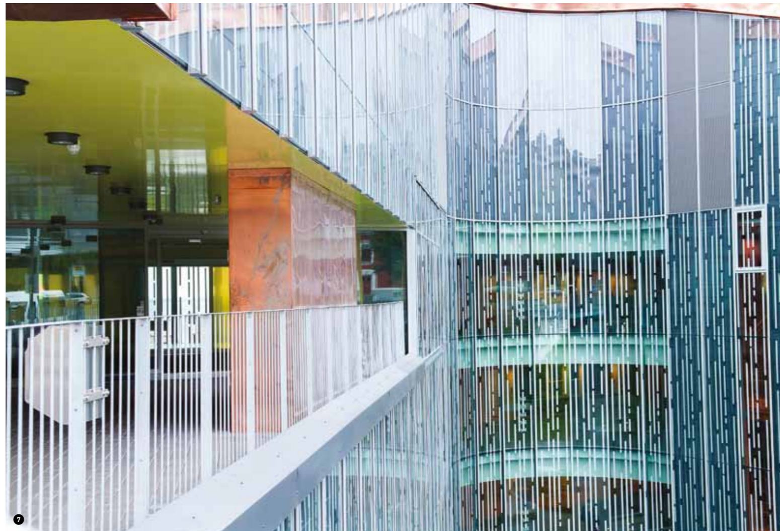
7 Tipotie, Tampere, Finland Our DALI router system controls lighting in the spacious multi-floor lobby.
