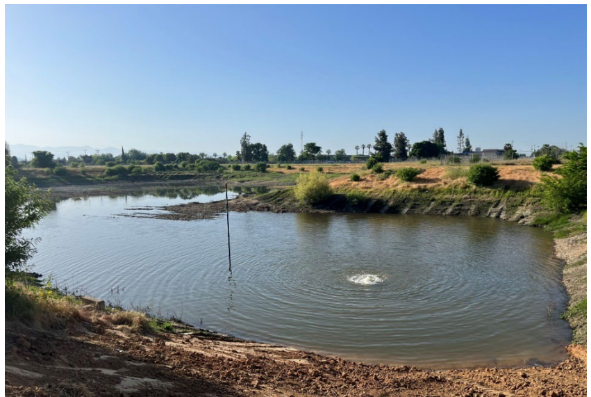
First flows into Lindsay Recharge Basin occurred in spring 2023.
