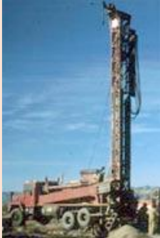
Figure 13.17 Typical borehole drilling equipment.
