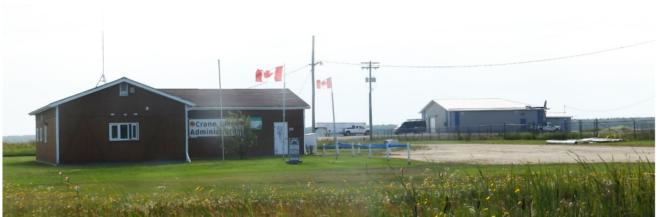
Crane River Water Treatment Plant to the right
