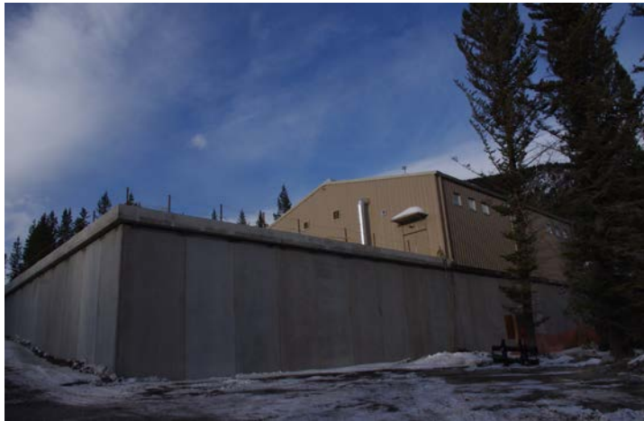
Figure 12. Water treatment plant located on top of treated water storage.
