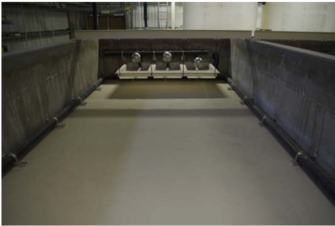
Figure 15. Filter cell before commissioning.
