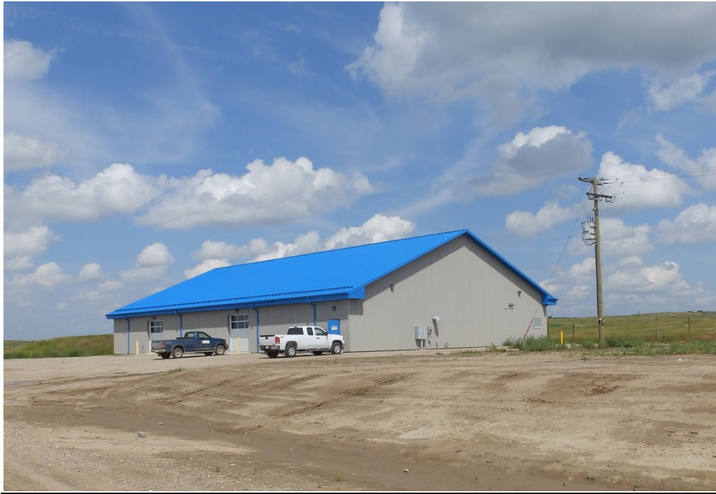
Figure 19. Exterior of WTP3..
