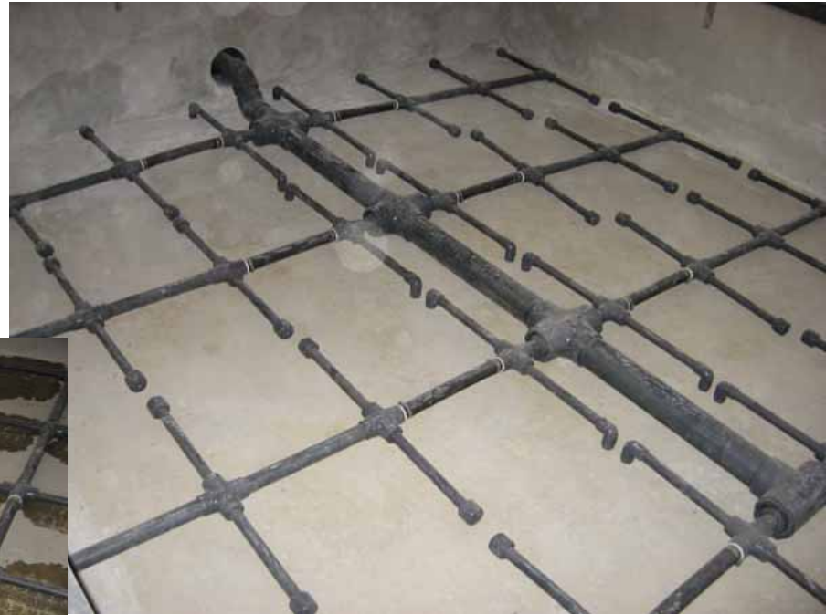
Testing the underdrain.
