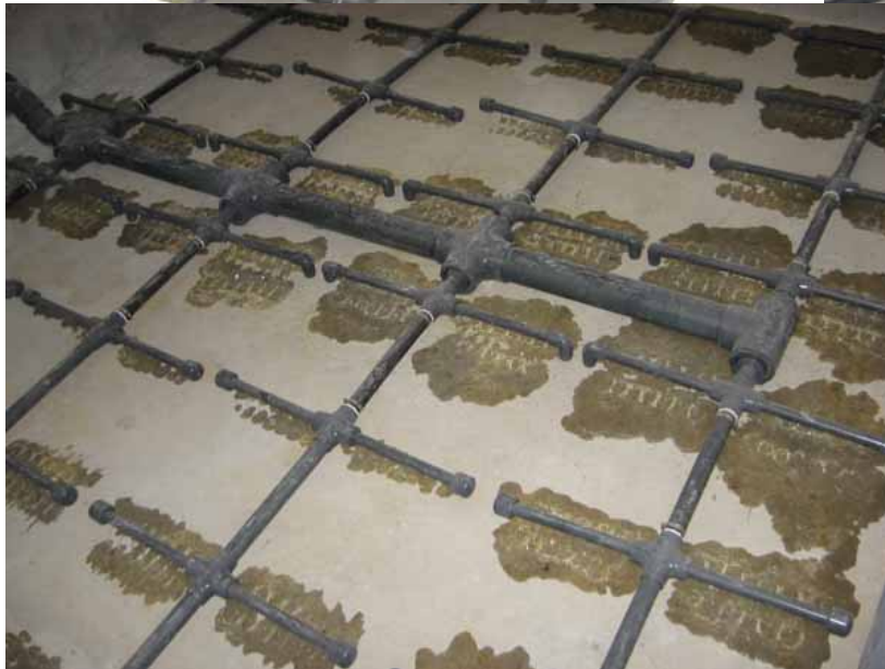
Testing the underdrain.
