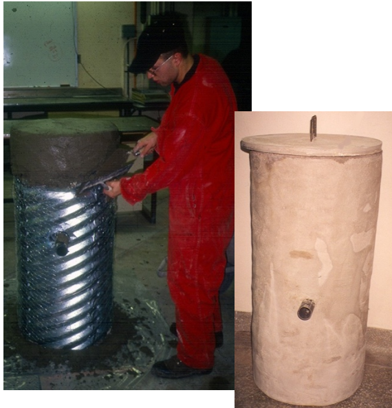
Ferro-cement construction of BioSand Water Filter at University of Calgary.
