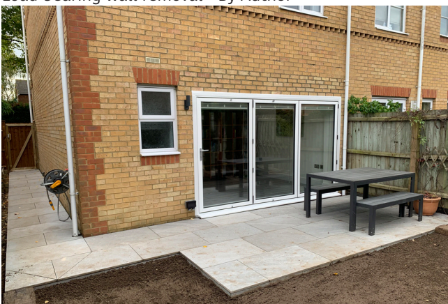
Load-bearing wall removal - By Author
