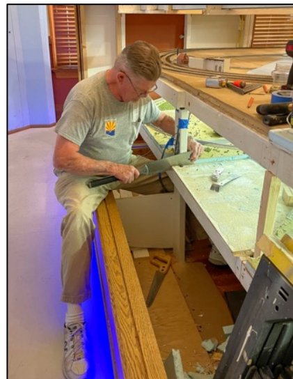
Ken Nelson begins construction of the support structure for the South face of the Grand Canyon.
