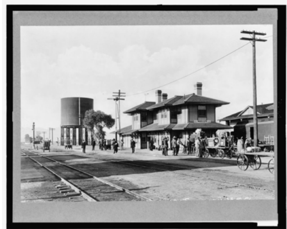
The Maricopa depot when it was the junction for trains to and from Phoenix, circa 1890.
