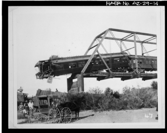
The 1902 Salt River Bridge collapse.
