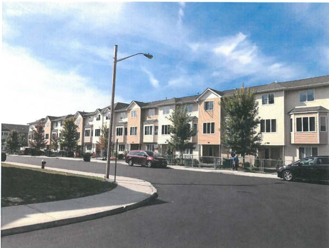
New Multifamily Housing, Zitomer Street
