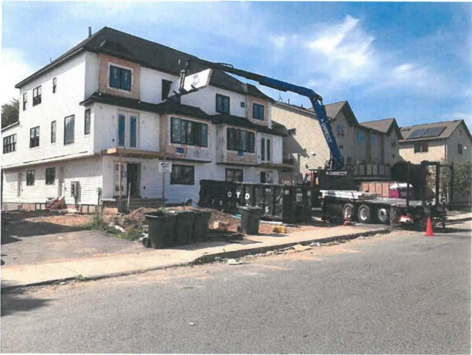
New housing under construction
