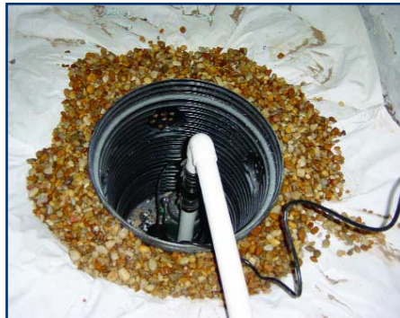
Use sump pumps if desired or when gravity drains are not feasible. This model includes a cap for the housing and an optional liquid water alarm to detect a failure of the sump pump system.
