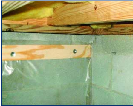
One way to mechanically attach a wall vapor retarder: secure it behind a preservative-treated plywood furring strip attached to the masonry with nails driven through washers. Photo credit: Bill Warren.
