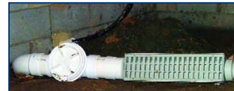
This crawl space drain and backflow valve assembly is ready for installation.
