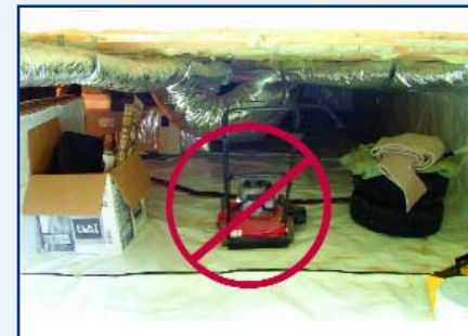
One of these items doesn't belong in a crawl space...
