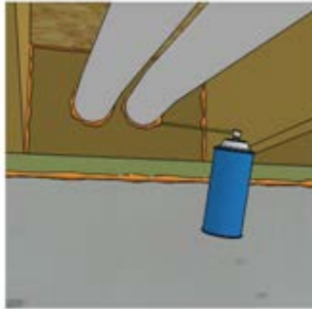
Figure 15. Foam sealant at band joist insulation and penetrations
