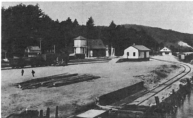
VIEW OF RAILROAD SQUARE FROM THE SOUTH
