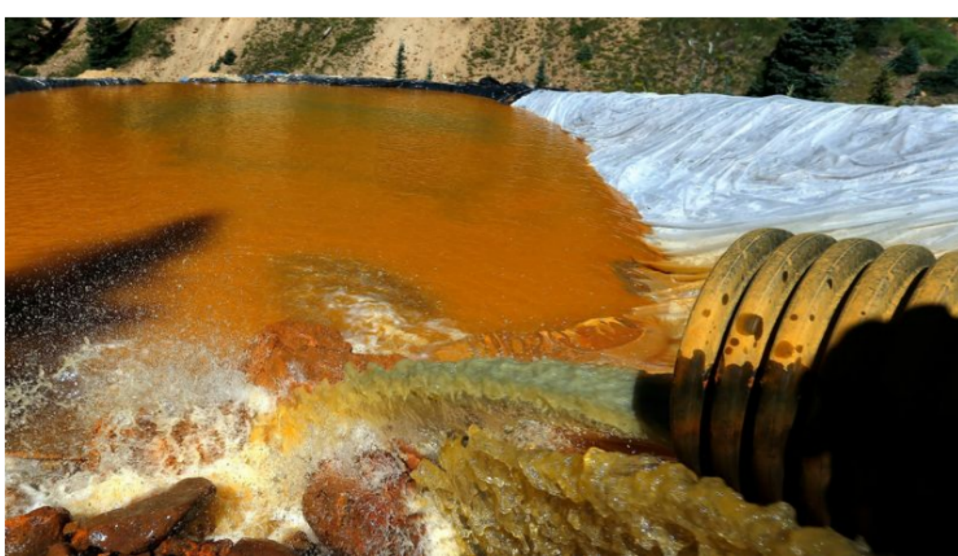
Orange-colored water in a retention pools built to contain the contaminated water that exploded from the Gold King Mine in 2015. (Brennan Linsley/AP)
