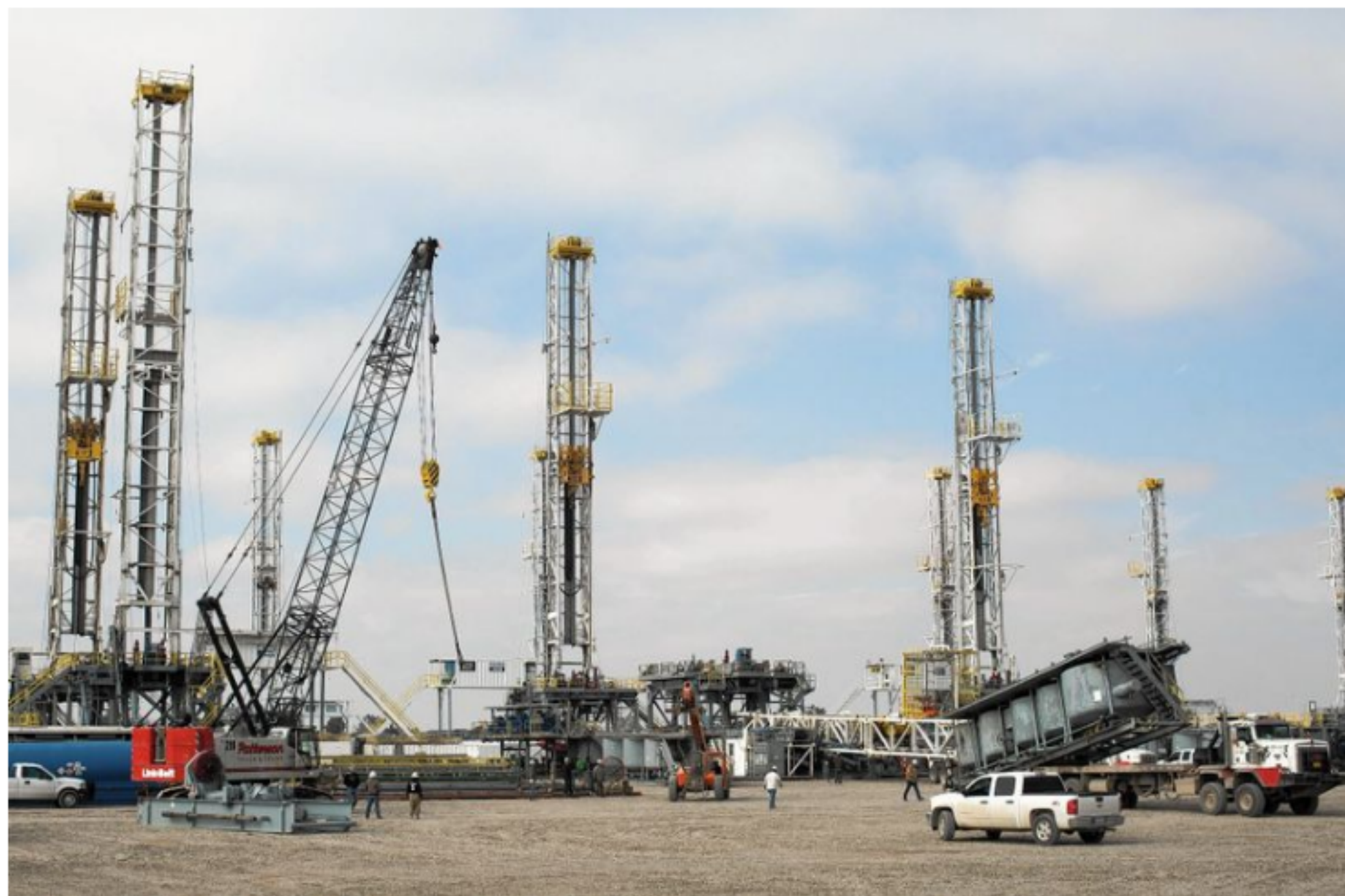
Oil drilling rigs sit idle in the West Texas town of Odessa. (Courtney Sacco / Odessa American)
