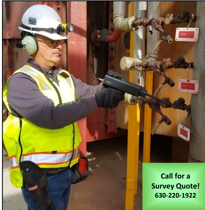
Bill Holub Conducting a Steam Trap Survey
