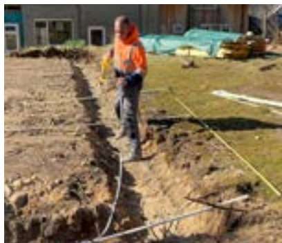
Measuring out the foundations
