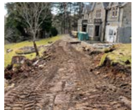
Creating the new drive way
