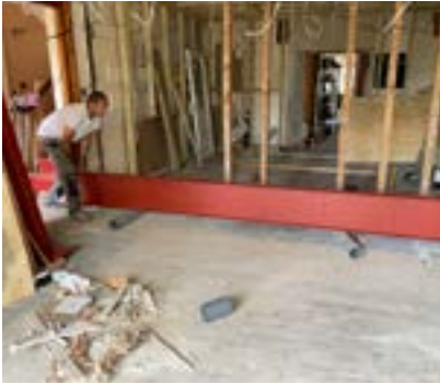
Installing the 4.5m RSJ
