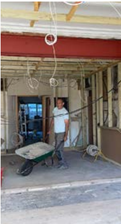
Installing the 4.5m RSJ
