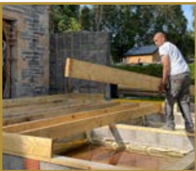
Building the floor for the extension
