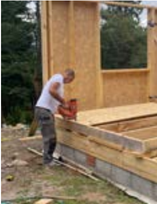
Building all the kits on site
