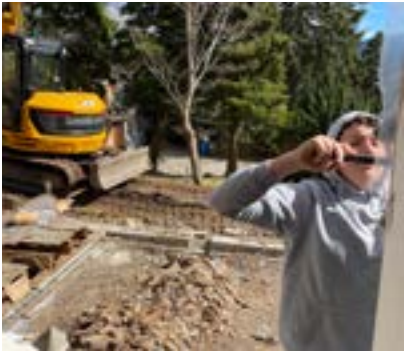
Anthony demolishing a wall
