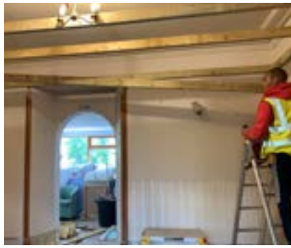
Framing the new ceilings
