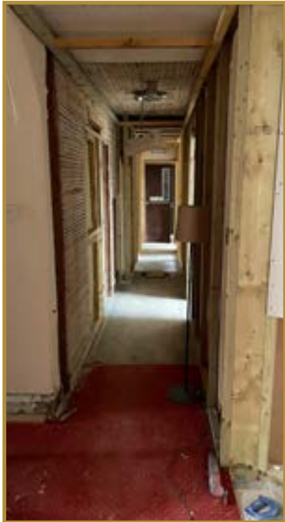
Lining the corridors
