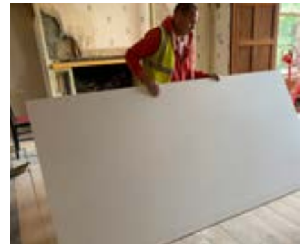
Over 100 sheets of plasterboard carried in
