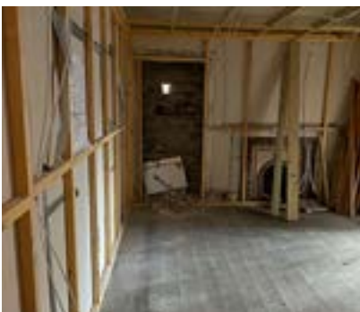
Lining all the inner walls
