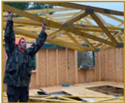
The trusses going up
