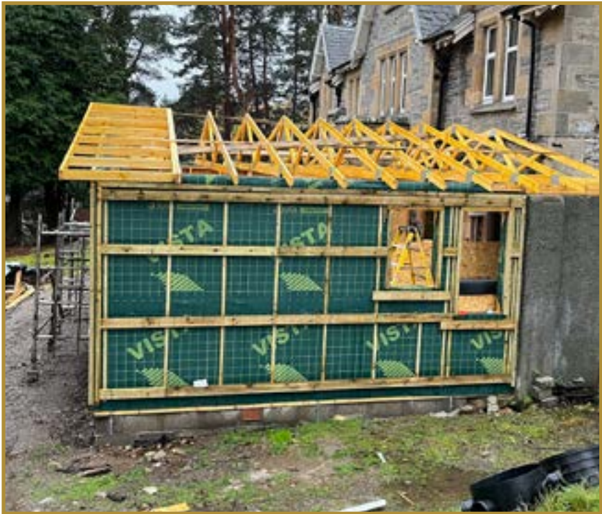
The extension with the trusses installed
