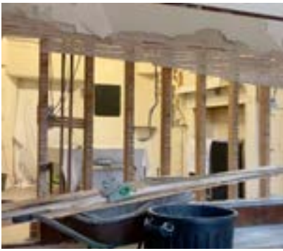
Removing the wall of the old kitchen
