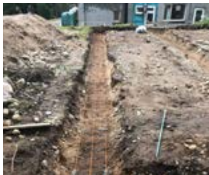
Preparing the foundations trench
