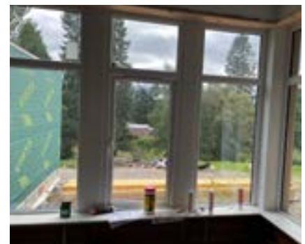
Over 50 new windows installed
