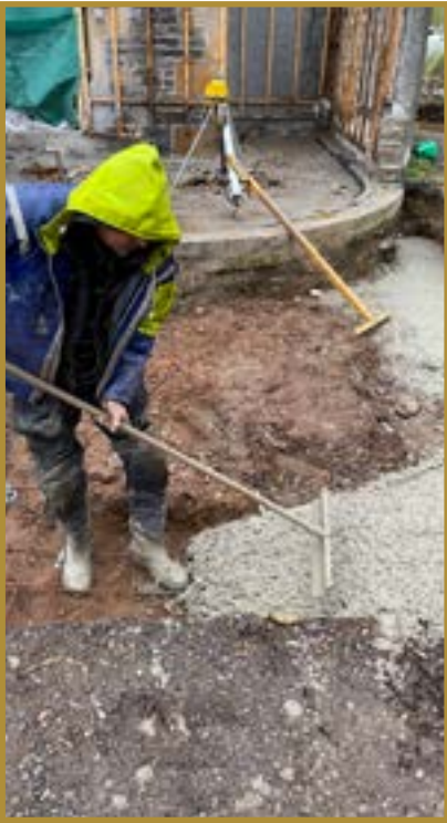
Nick laying the concrete for the extension
