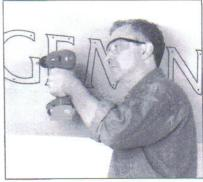
3. Drill 1/4" holes 3 inches deep where indicated on your template. Remove the template and clean out all drill holes using any of the following methods: a quick puff of air; using the vents on your drill; compressed air or a turkey baster.
