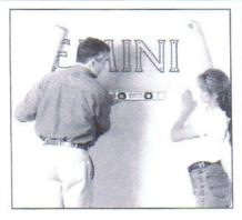
Tape one edge of the template to the installation surface with masking tape and unroll it. Level the template and tape the other edge to the installation surface.
