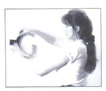
6. Push the letter into the drill holes using a shim to assure the proper standoff of the letter from the wall. Repeat steps 3 through 5 for the rest of the letters.
