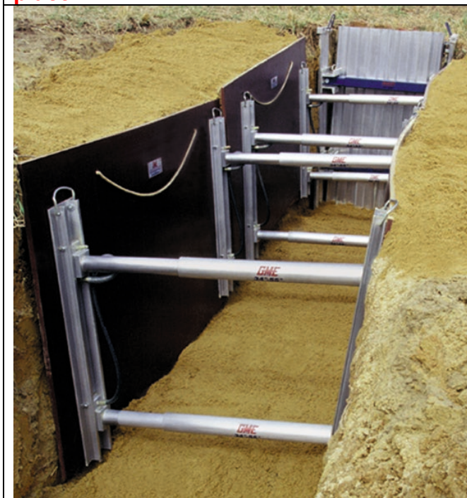
Hydraulic jacks holding trench shielding in place
