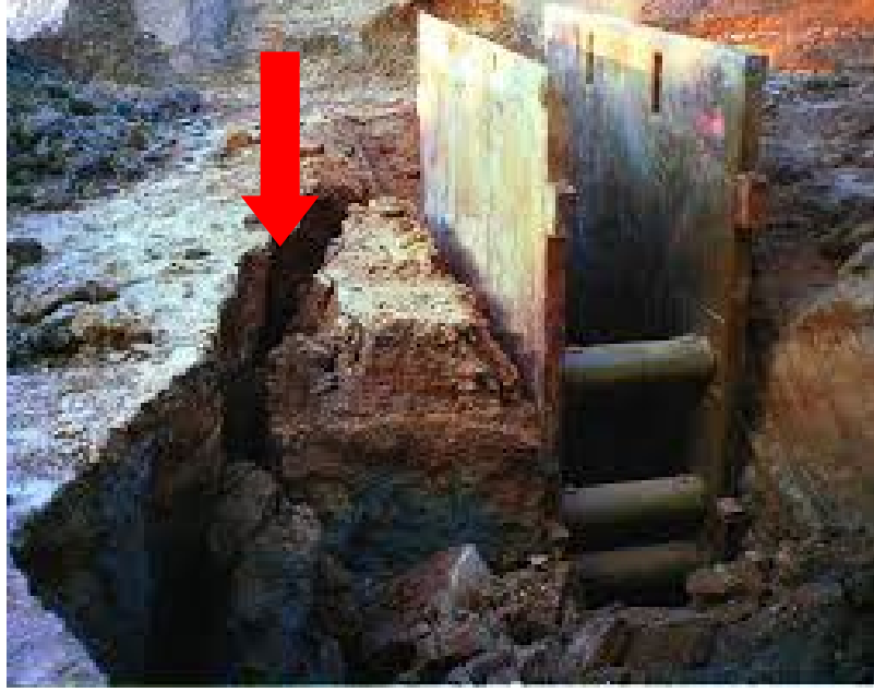
The importance to use a trench box on our job sites
