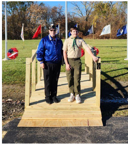
Commander Tim Shosey Post 4 and Matthew Oliver Troop 1402 Fraser, at his Eagle project, which was constructing a bridge that crosses a ditch to our new Flag poles. The bridge will be used for our Memorial programs.
