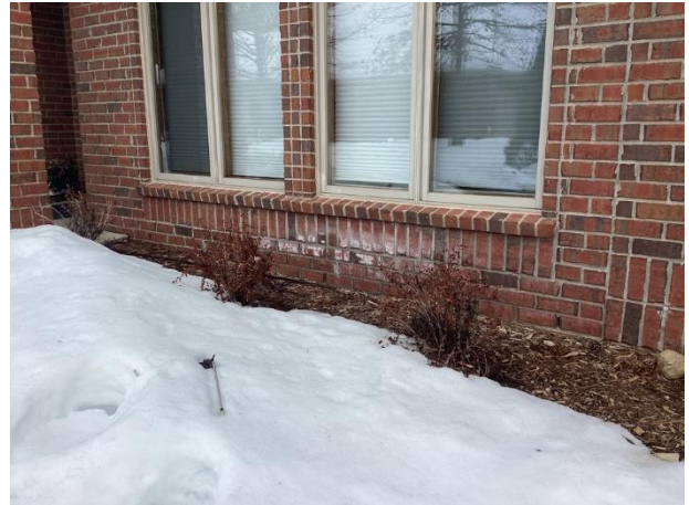
Efflorescence
