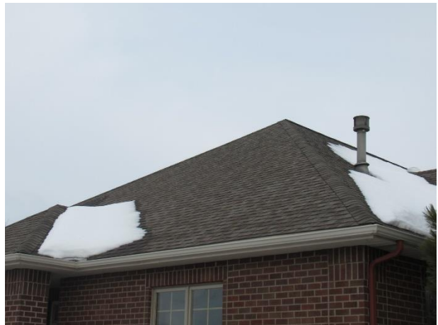
Asphalt shingle roof overview
