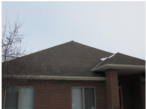
Asphalt shingle roof overview
