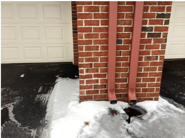
Previous mortar repair
