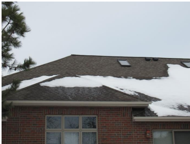
Asphalt shingle roof overview
