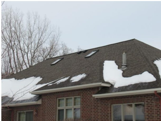
Asphalt shingle roof overview
