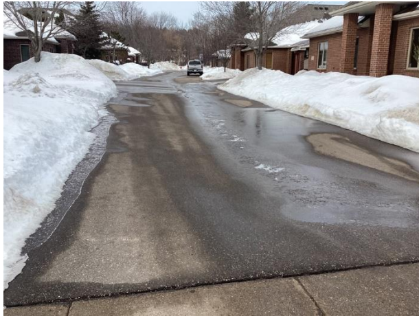
Repaved access drive and driveways
