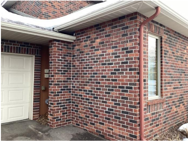
Masonry façade overview
