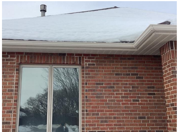
Previous mortar repair
