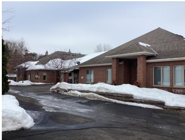
Building exterior overview
