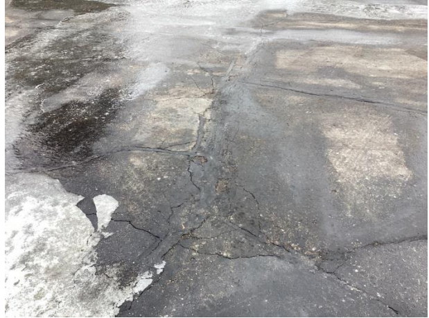
Fatigue cracks
