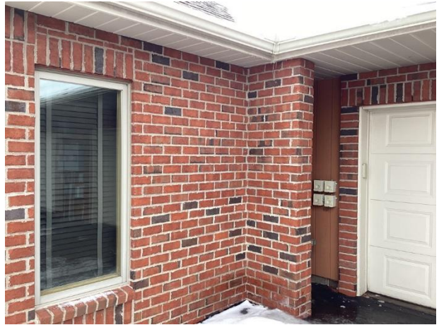
Masonry façade overview
