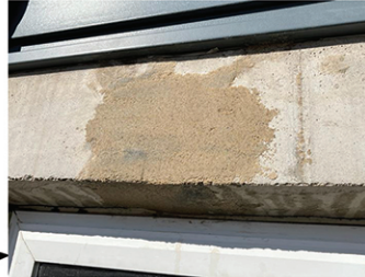
With CONCRETE FUSION Crack Repair Product
