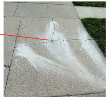
Staples put in place before filling crack.
