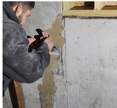
We patch with CONCRETE FUSION Crack Repair Product
