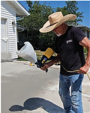
You spray our mix to cover all the crack lines.
