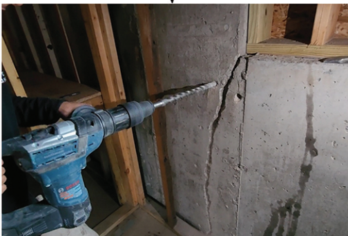
We drill holes for our Staple System
