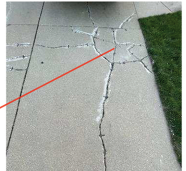
Staples put in place before filling crack.
