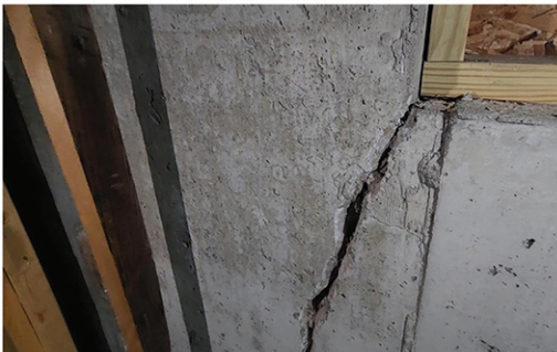
Foundation Crack
