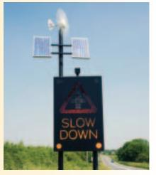
**Solar energy** is sometimes used to power road signs. Photovoltaic cells use the photoelectric effect to convert the energy of light into electric energy.
