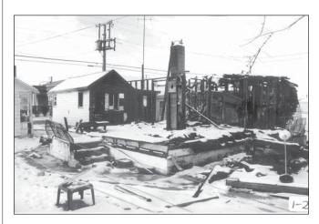
Figure 1 – Wood Frame Home Remains after Natural Gas Explosion
