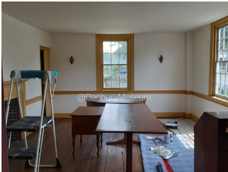
The Rider House dining room with a fresh coat of paint.
