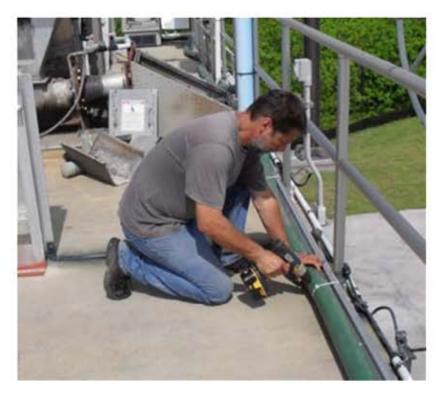
Secure hose with zipties and drill 1/4" holes, evenly spaced, facing the odor source.
