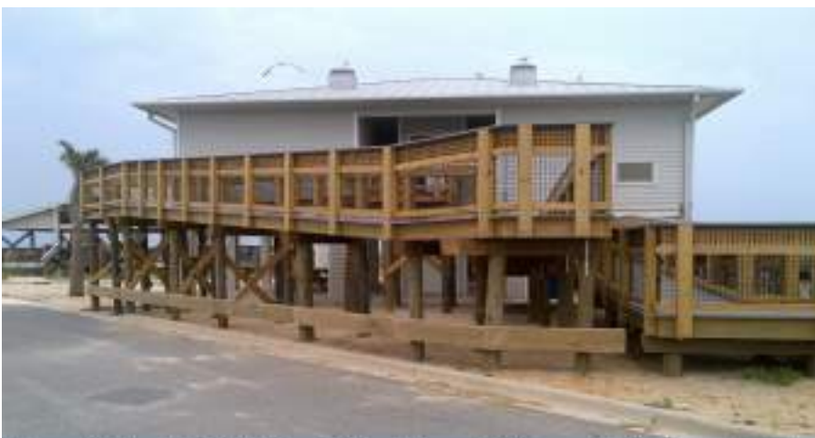
Figure 3. Florida, Gulf Coast, flood Zone V. Ramp built after original elevator determined to be unsustainable due to significant maintenance problems.
