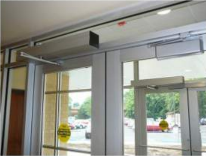
Power door operators (left doors), door closer (right door). Photo courtesy Hager Companies
