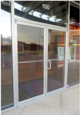
Pivoted door Photo courtesy Allegion
