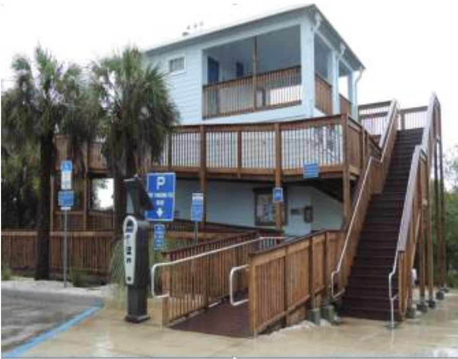
Figure 1. Florida, flood Zone V. Ramp wraps around entire building. Has composting toilets, battery and solar electric system, emergency plan requires pumping out tank and filling with clean water.
