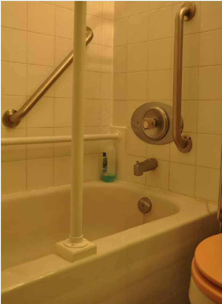
Figure 2. Demonstration set up of both conventional grab bars (nominally meeting the length and location criteria of proposed IRC requirements and a stanchion plus a horizontally-fixed section—like a handrail—of the same tubing used for the stanchion (both completely meeting the length, location and structural strength requirements of proposed IRC requirements (which are consistent with IBC, ICC A117.1 and NFPA requirements)
