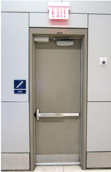
Electromagnetic door lock (top-left corner of doorway) and door closer. Photo courtesy Allegion
