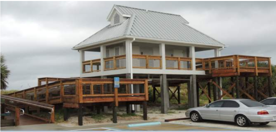
Figure 4. Southwest Florida, flood Zone V. Extensive ramp wraps around three sides.
