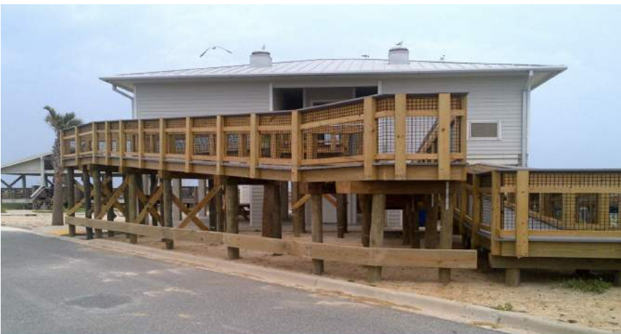
Figure 3. Florida, Gulf Coast, flood Zone V. Ramp built after original elevator determined to be unsustainable due to significant maintenance problems.
