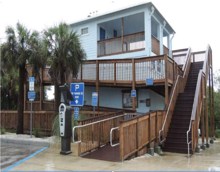
Figure 1. Florida, flood Zone V. Ramp wraps around entire building. Has composting toilets, battery and solar electric system, emergency plan requires pumping out tank and filling with clean water.
