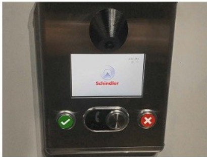
The device gives riders the option to communicate visually by answering on-screen questions.
