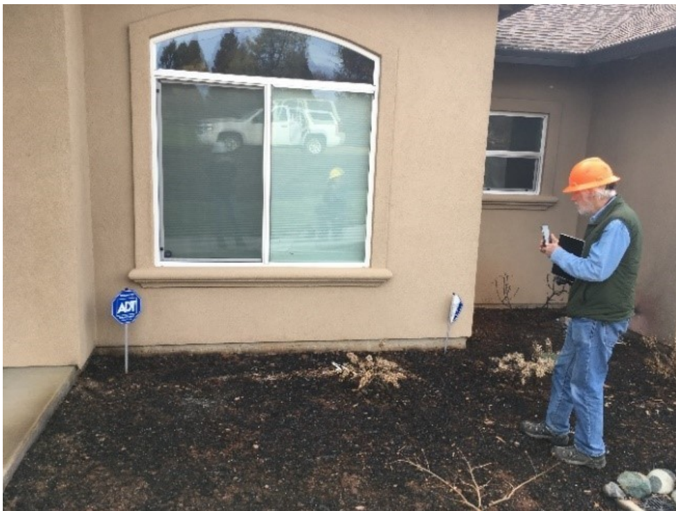
Failure of the outer layer of a double-glazed window
